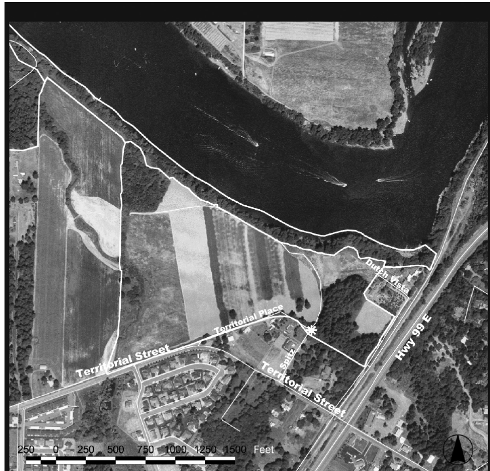
Figure 2-5. Existing access and roads, Fish Eddy
