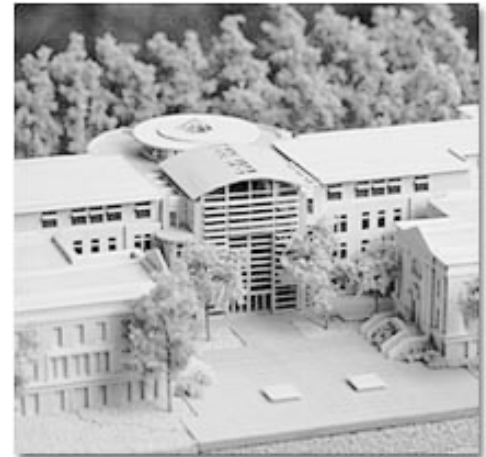
The new business school addition will require half the energy of a typical campus building. Passive ventilation and cooling strategies are integrated into the design.
