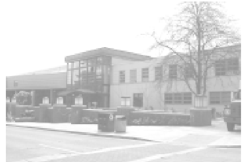
The new recreation center which included a significant remodel of the former PE complex demonstrates the cultural, environmental and energy saving benefits that occur when priority is given to maintaining and renovating existing buildings.
