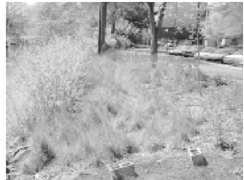
A bioswale filters runoff from a parking area (right) and delivers it to an open water way (left). Plant material and terrain slow and absorb runoff, filter sediments, and facilitate infiltration. When appropriate, we consider overland flows and ponds to temporarily impound water and allow a slower rate of infiltration.
