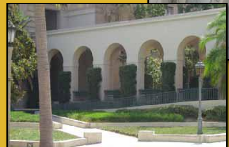
*Reconstruction: historic arcade after demolition for base isolators
