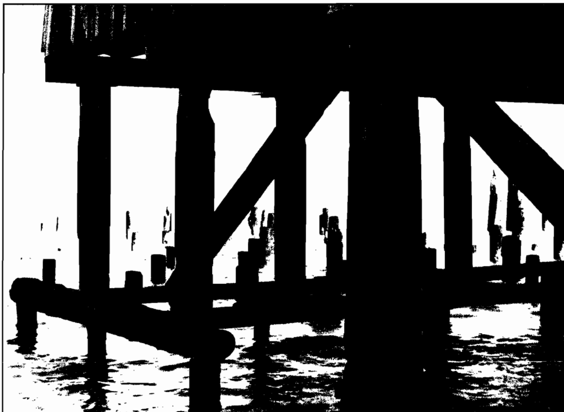
Figure 15. Cannery pilings and substructure. Source: CCHS
