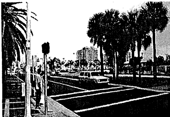
Well-Marked Crosswalk with a Pedestrian Signal (Bal Harbour)
