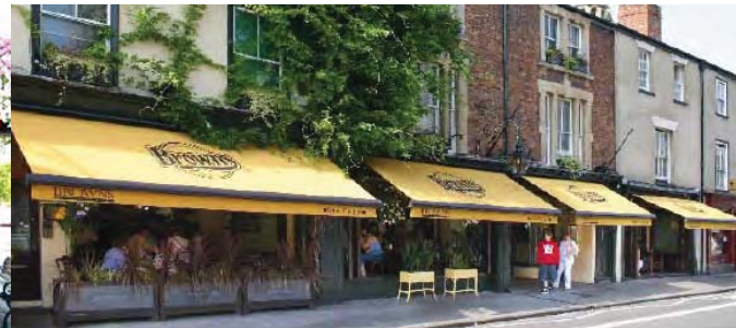
continuous overhead weather protection
