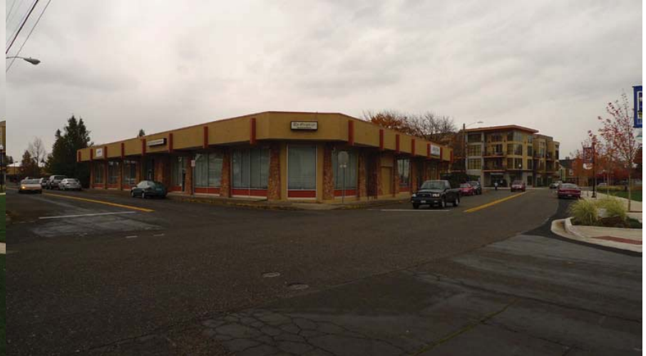
3rd and Hood - existing buildings on site
