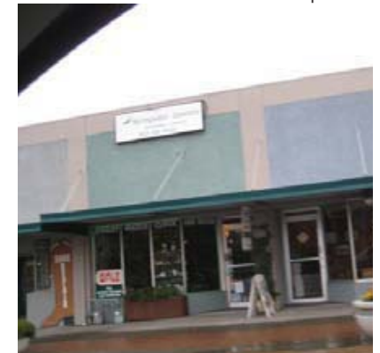
strip facades and surface parking
