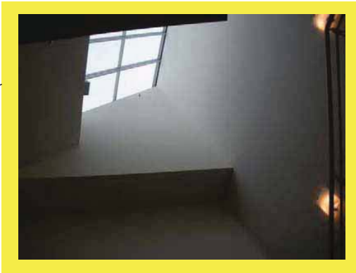
skylights add daylight in stairwells
