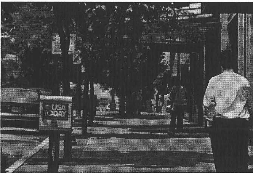
Figure 4. Sidewalks should be properly maintained, free from obstructions and potential problems for pedestrians.
