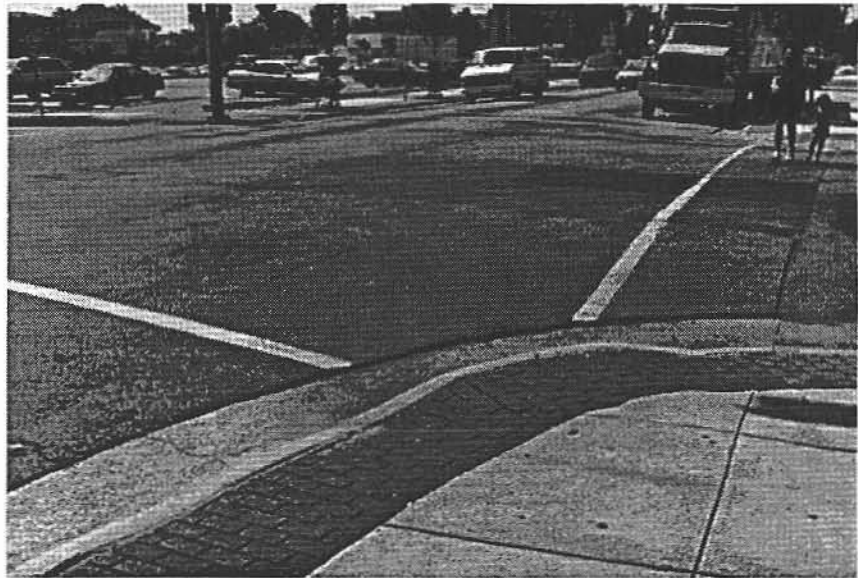
Figure 2. Curb cuts are the single most important design consideration for persons in wheelchairs.
