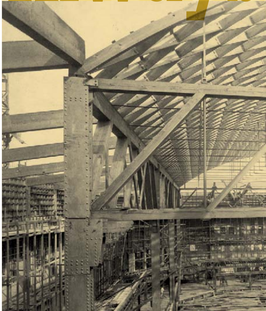
ABOVE: The steel and wood framework of Mac Court during construction in 1926. TOP RIGHT: Clifton Nesmith McArthur '01, for whom Mac Court was named, is at far right. McArthur, who was the first president of the student body and student athletic director, later served as speaker of the Oregon House of Representatives and as a congressman. BELOW: an ivy-covered Mac Court overlooking a 1947 baseball game at Howe Field.
