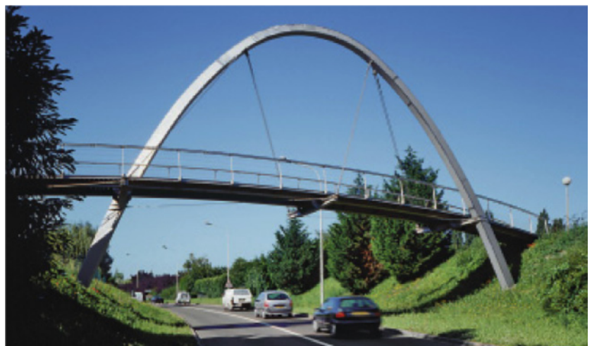
Figure 38: Example of a Pedestrian Overpass.
