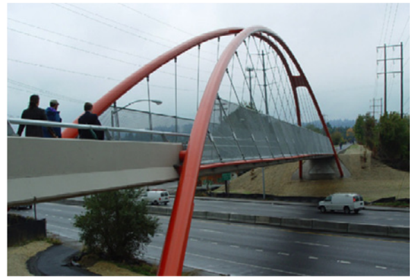
Figure 36: McLoughlin Pedestrian Bridge, Portland.
