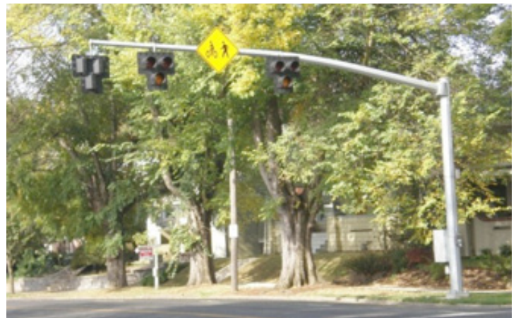
Figure 21: HAWK Signal as Seen by Motorists.
