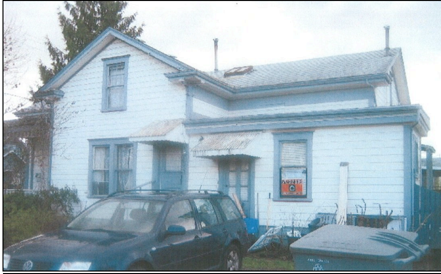
Figure 5.11 Gray House Exterior Showing Windows to be Restored and Siding to be Scraped and Painted, 2007. Source: Special Assessment Files, State Historic Preservation Office.
