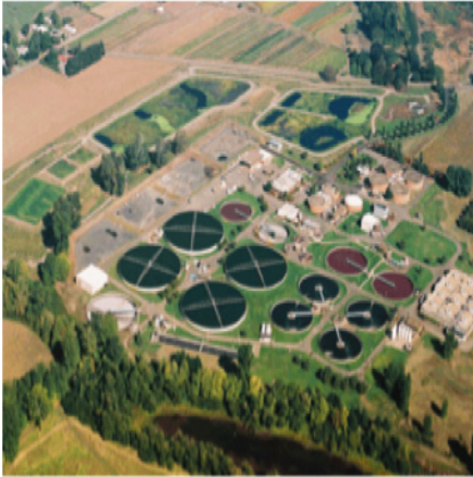
Figure 1: Willow Lake Water Pollution Control Facility
