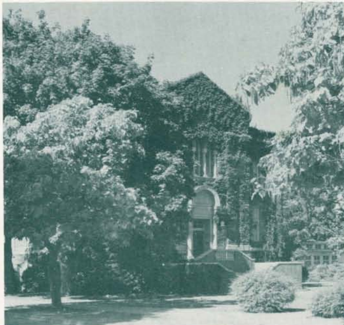
Oregon Building, headquarters for the College of Liberal Arts.
