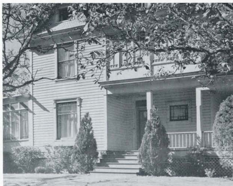
The structure known as Canard Club, the "House of Characters," which fell victim to wartime conditions, now houses married students, mostly veterans.
