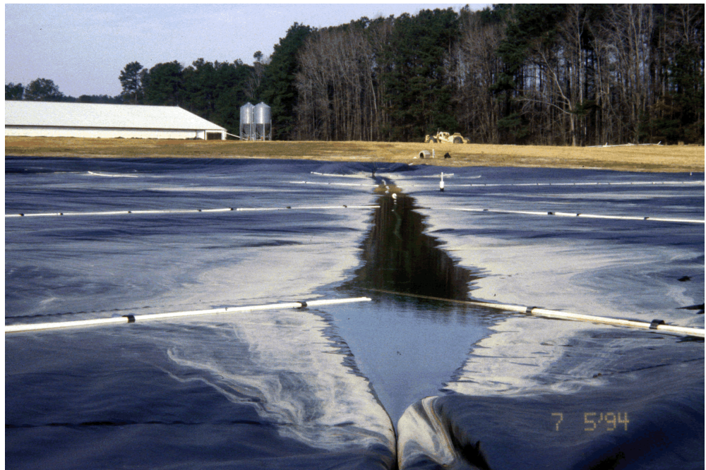
Figure 2. Covered lagoon digester
