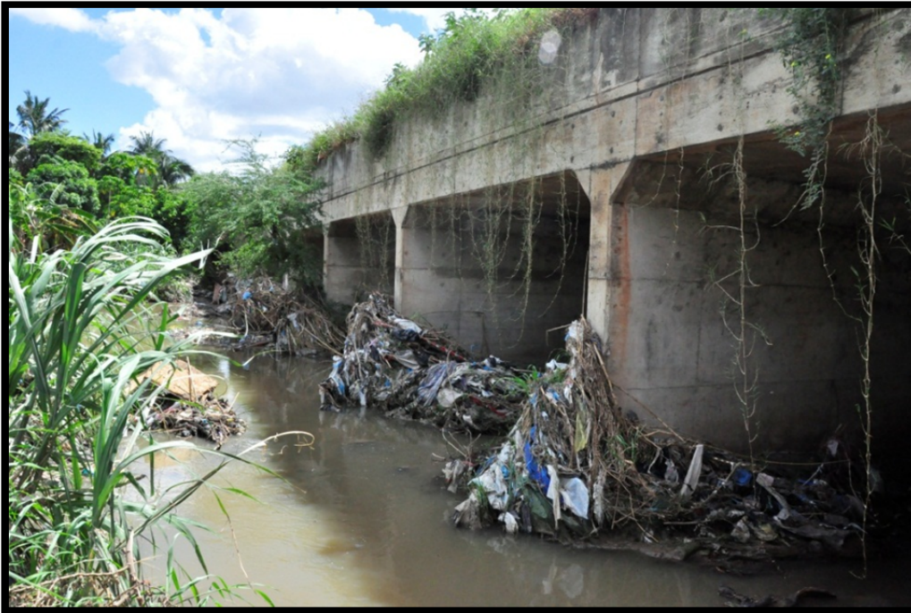
Figure 4.9. Trash buildup on the Msimbazi river. This picture is taken from one of the plots in the Msimbazi Valley. The bridge goes under Kawawa Road, a major thoroughfare in the city (A. Halloran).
