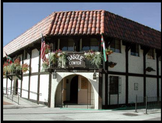
Figure 4.3. Basque Center located at the corner of 6 th and Grove Street, Boise, Idaho resembles Basque Country baserri -farmhouse architectural style. Source: Thebasqueblock.com, 2012.
