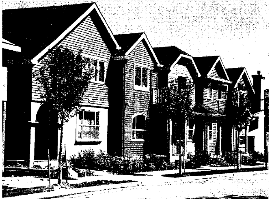
The village contains several house types to appeal to a wide spectrum of potential buyers. The rowhouses meet the needs of a growing market segment seeking economy and ease of maintenance, and are priced from $134,500 to $290,000 to appeal to a variety of income levels.
