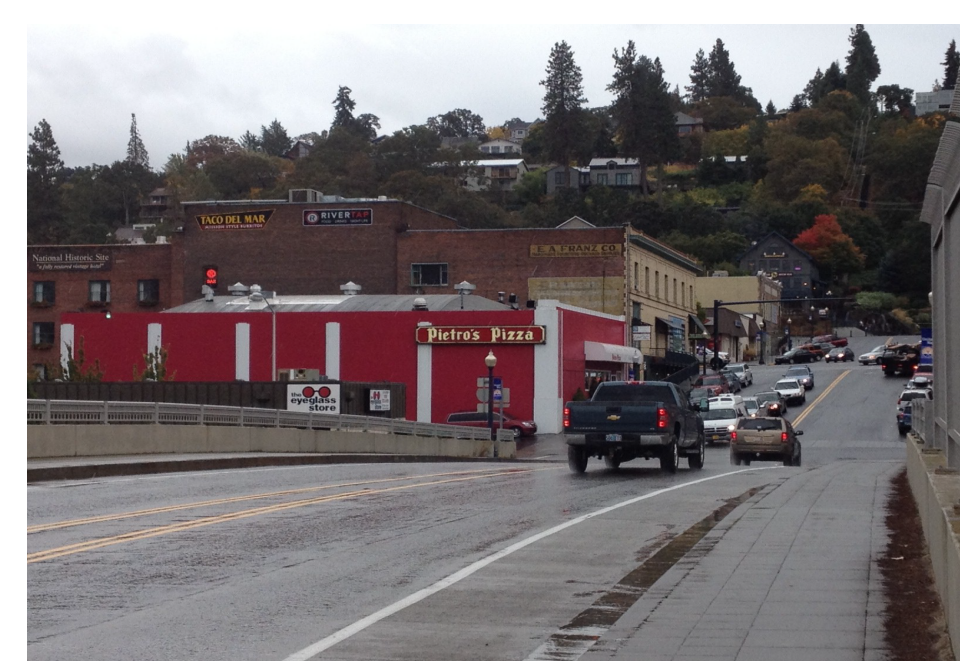
2ND STREET APPROACH // EXISTING CONDITION
