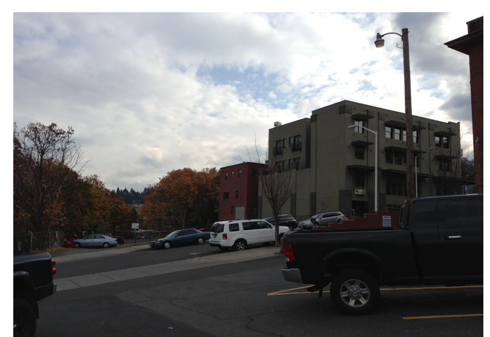
TOWER LOCATION // EXISTING CONDITION
