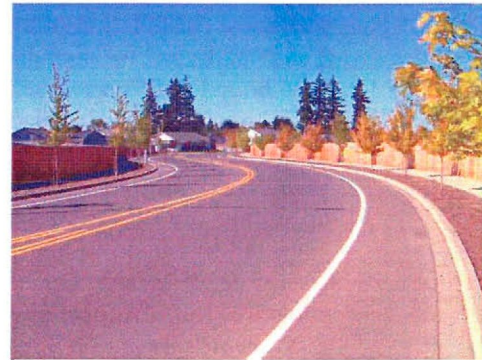
Suburban collector road through residential area with bike lanes, landscaping and sidewalks.
