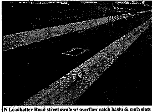
N Leadbetter Road street swale w/ overflow catch basin & curb slots
