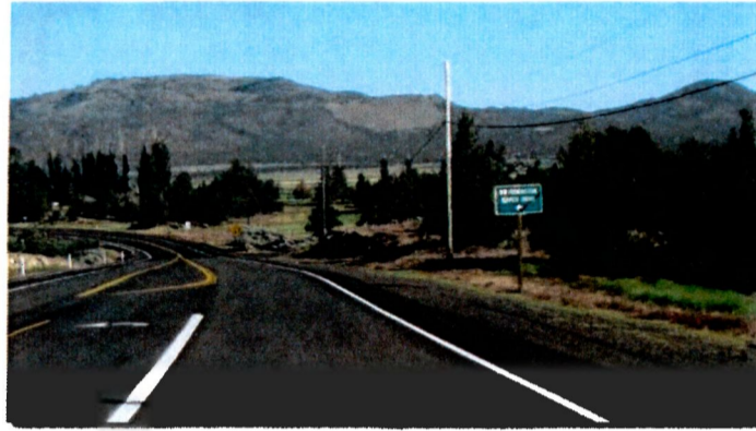
Exhibit 4-3 Existing shoulder along OR Highway 126 with rock outcroppings, utility poles, and guardrail within the clear zone.
