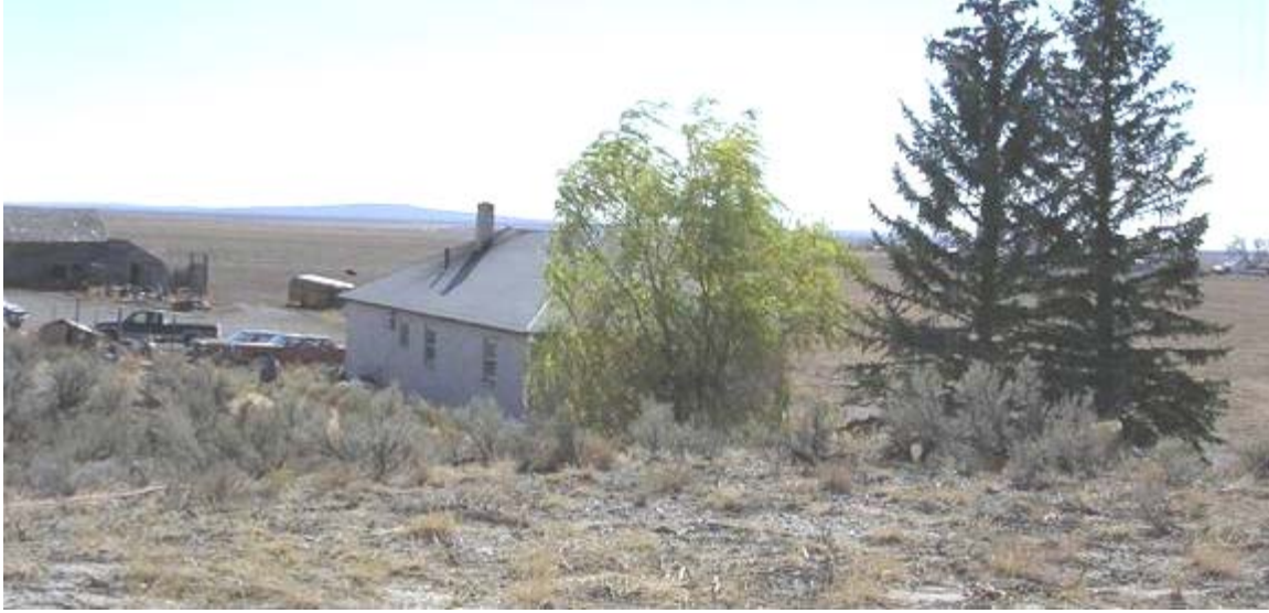
Figure 21. Dwelling along 2900 West with hazardous fuels within 10 feet of structures.
