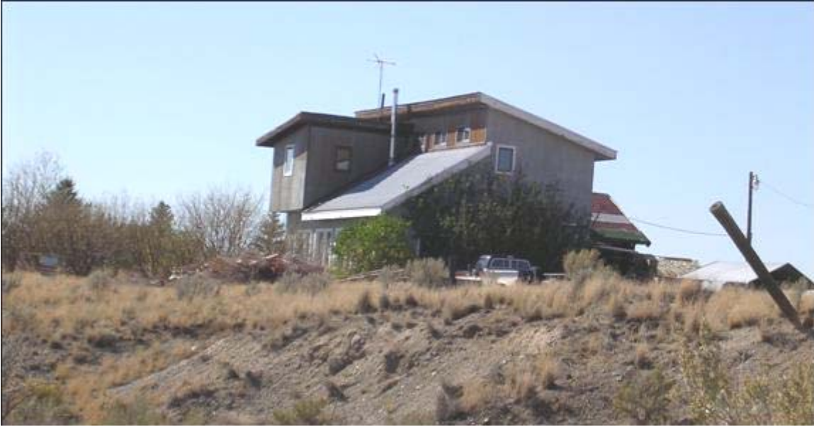
Figure 23. Single-family dwelling approximately 2 miles southwest of Butte City. This home is along 2150 North and shows an overhanging roof and landscaping and native vegetation (sagebrush-grassland) growing within 10 feet of structure.
