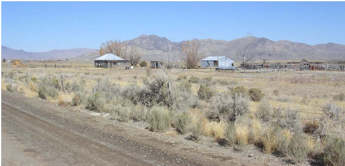
Figure 20. Dwelling along 2900 West with hazardous fuels near structures.
