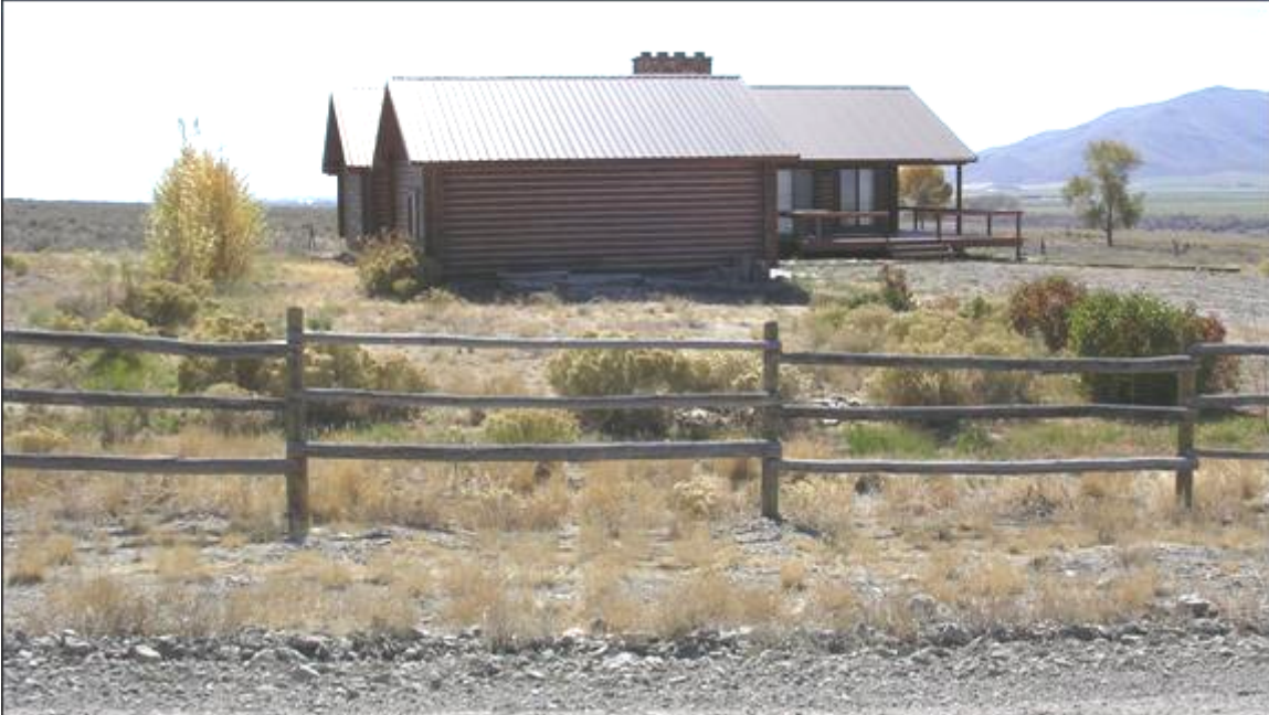
Figure 16. Single-family dwelling showing good fire prevention measures.
