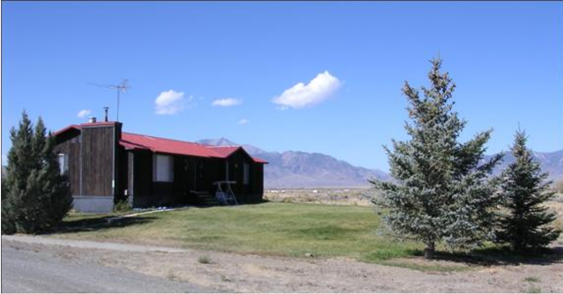
Figure 14. Single-family dwelling at 3556 US Highway 93. This home exhibits good fire prevention measures including a metal roof and 50 feet of landscaping between the home and the wildland-urban interface.
