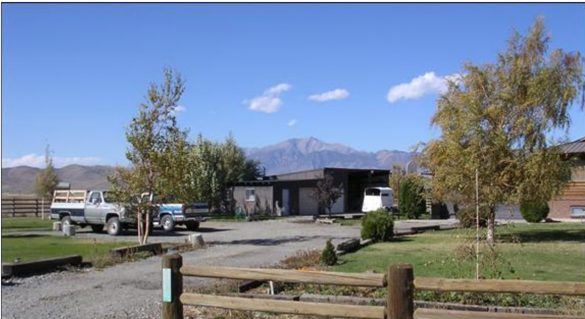
Figure 15. Single-family dwelling 3.5 miles north of Moore at 3592 W 3690 N. This home exhibits good fire prevention measures including a metal roof and 50 feet of landscaping between the home and the wildland-urban interface.
