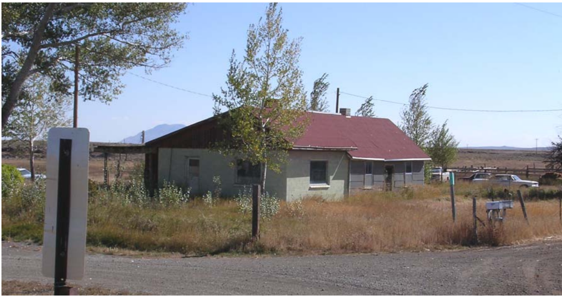
Figure 22. Dwelling along 2900 West with hazardous fuels within 10 feet of structure.
