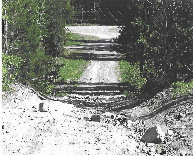
Figure 19: Suitable fuel break between improved property and WUI (south border of Silverhawk SD).
