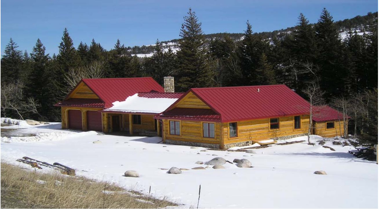
Typical new interface area construction--log with metal roof
