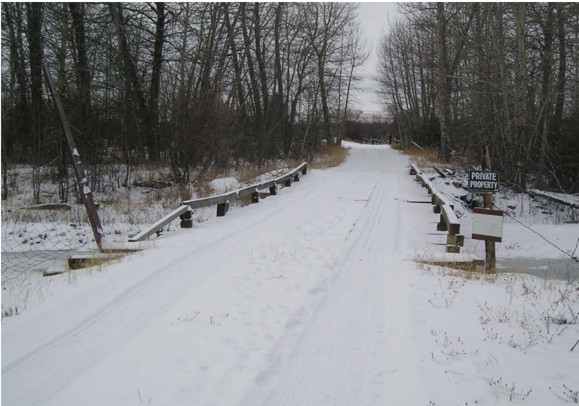
Access across Rock Creek to Western Ranch Estates Subdivision
