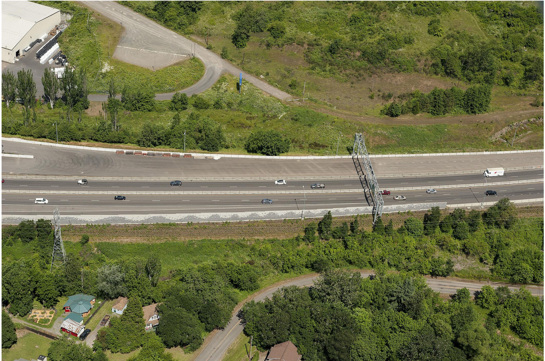
South section of the southbound sound wall (facing east)
