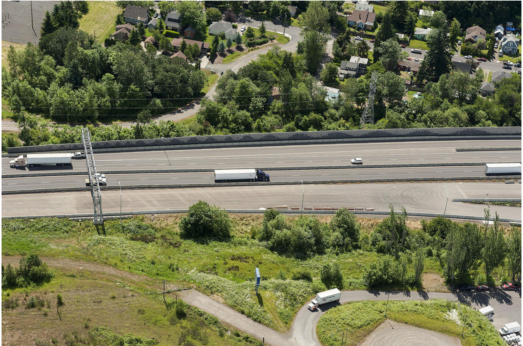
South section of the southbound sound wall (facing west)
