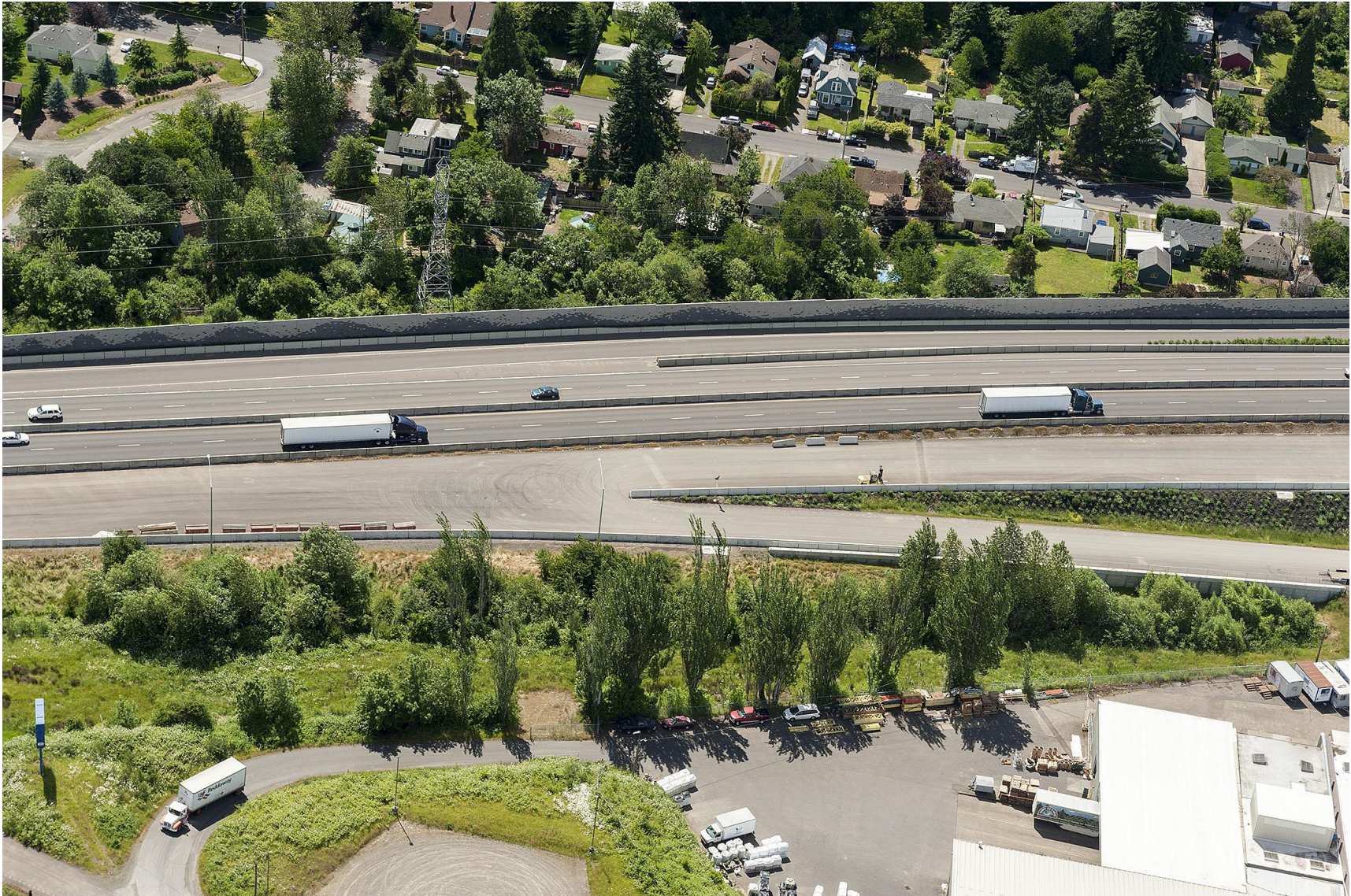
Mid-section of the southbound sound wall (facing west)
