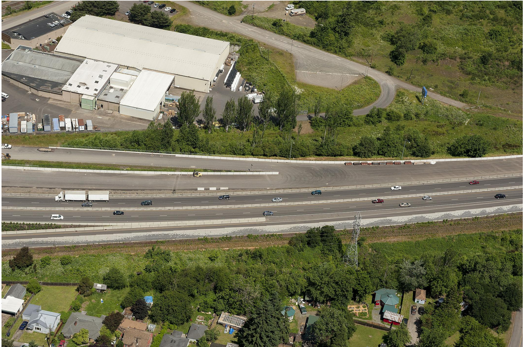
Mid-section of the southbound sound wall (facing east)
