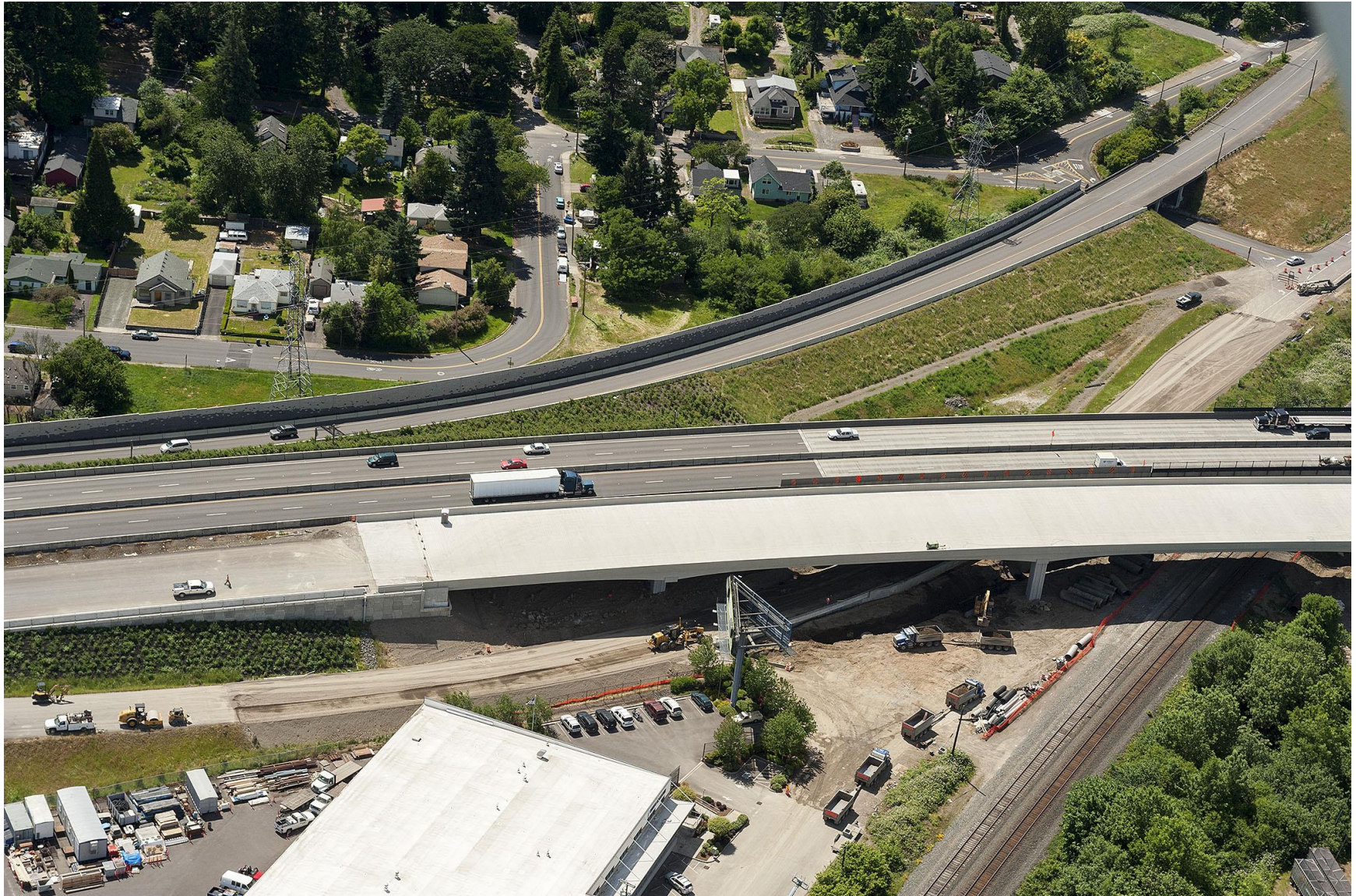
Northwest section of the southbound sound wall (facing west)
