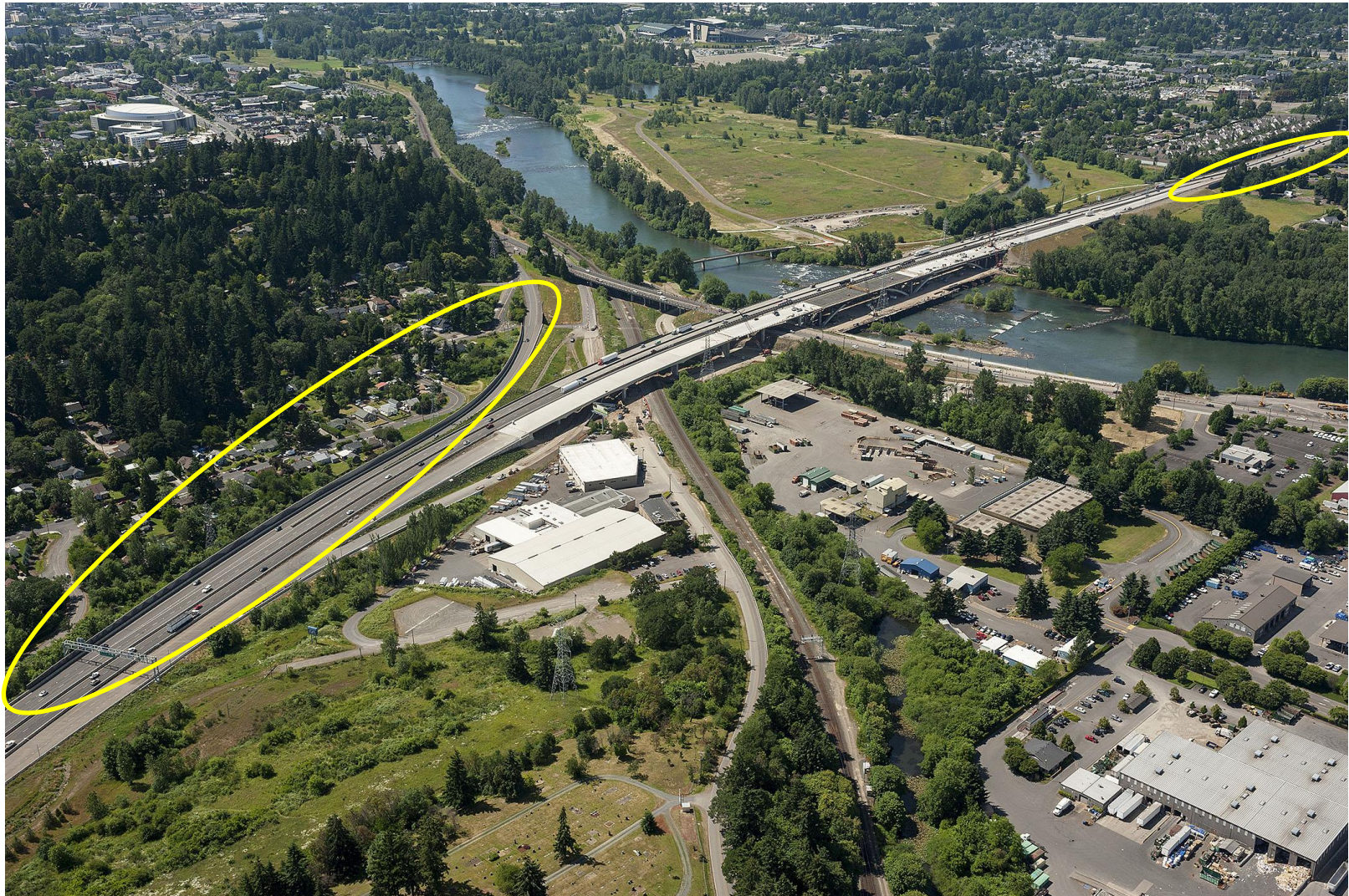
The entire Willamette River Bridge Project (facing west/northwest) [southbound sound wall (highlighted left) and northbound sound wall (highlighted right)]
