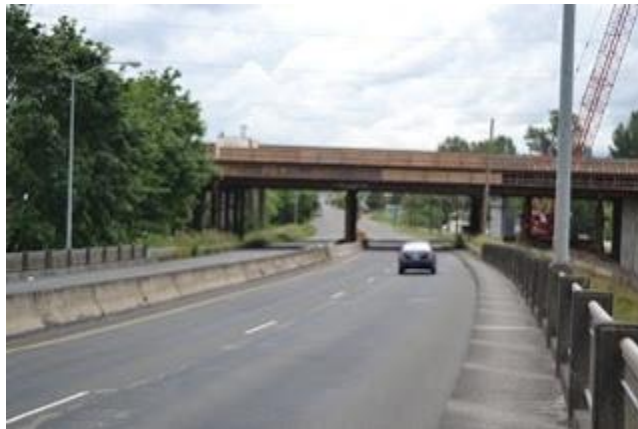
Bridge falsework over Franklin Boulevard.
