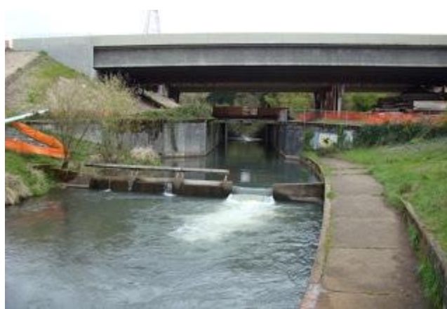
The Canoe Canal before we removed the walls.
