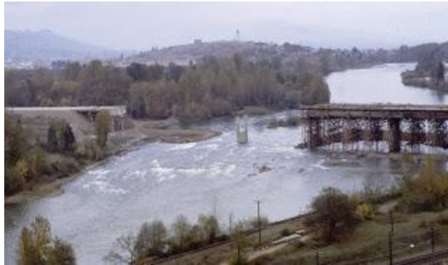
Construction of the original Willamette River Bridge circa 1960.
