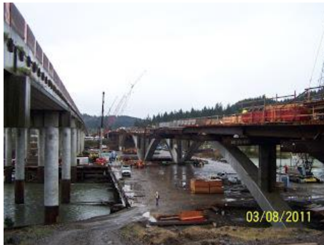
The work bridge supporting construction work and the new arches.
