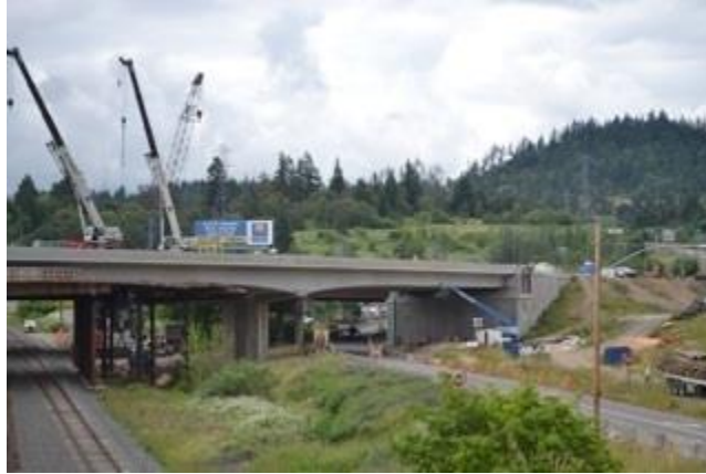
New bridge exposed south of Franklin Boulevard.
