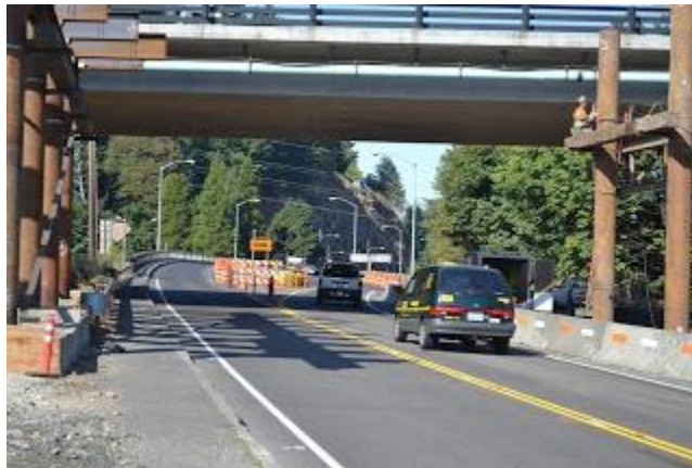
Westbound traffic returns to regular westbound lanes after passing under I-5.
