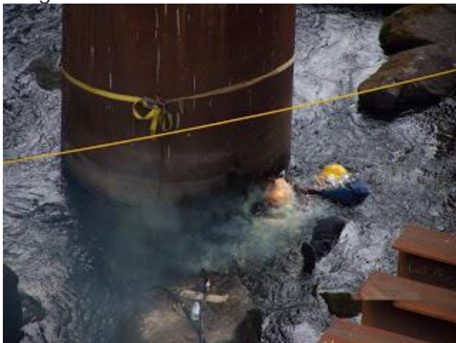
These pictures show crews placing a temporary bridge pier from the river onto the work bridge.
