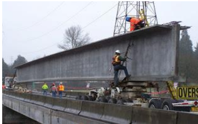
Workers prepare to unload a giant beam.
