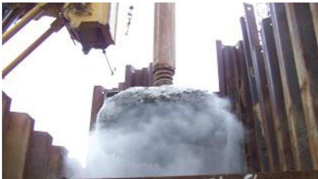
When crews first lower the drill into the target, they have to measure the distance from the auger to the walls of the shaft, ensuring that it is no more than three inches.
