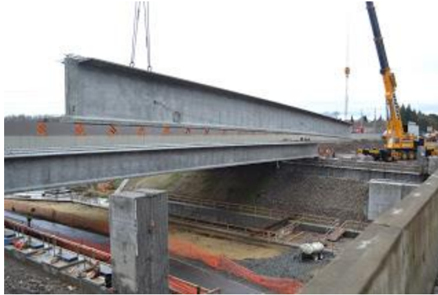
Large cranes carefully move the beam into place.
