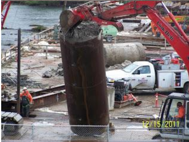
These pictures show crews placing a temporary bridge pier from the river onto the work bridge.
