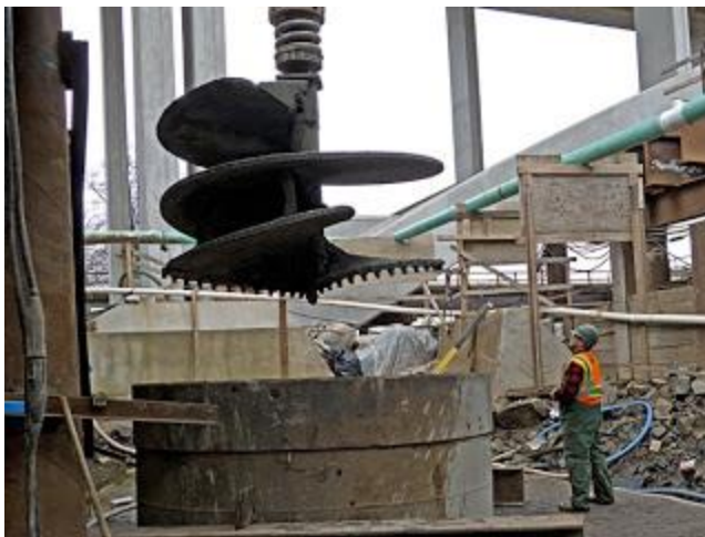
When crews first lower the drill into the target, they have to measure the distance from the auger to the walls of the shaft, ensuring that it is no more than three inches.
