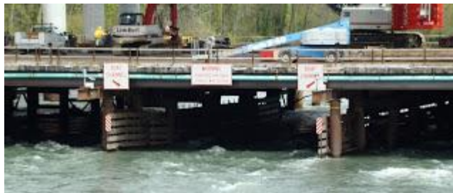
These signs show boaters where to pass safely under the workbridge.
