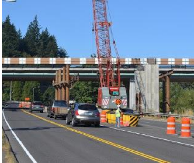
A flagger directs westbound traffic during pile driving and falsework construction.
