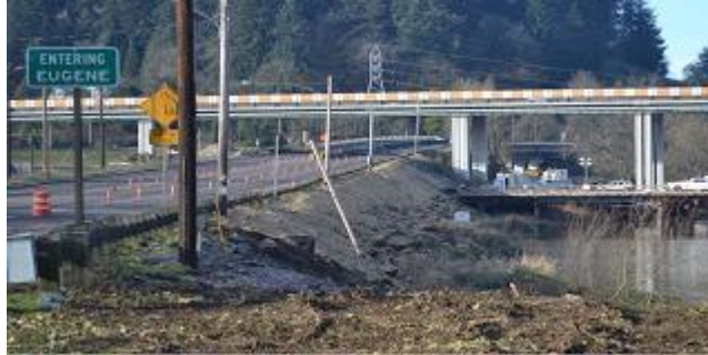
This view is looking west from upstream of the new I-5 bridge.
