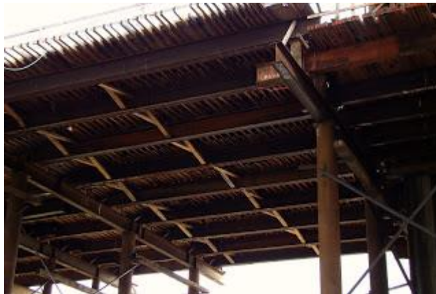
The steel supports and wooden falsework are still intact here.
