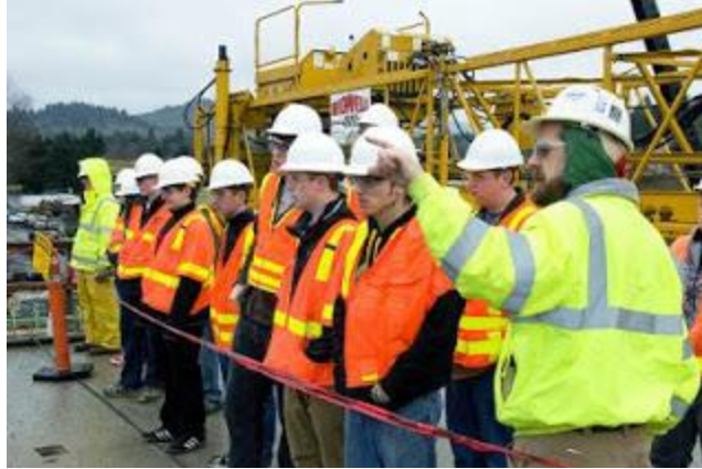
Above, OBEC engineer Brad Larsen (right) shows students how the large paving machine behind them built the concrete deck for the new northbound bridge.
