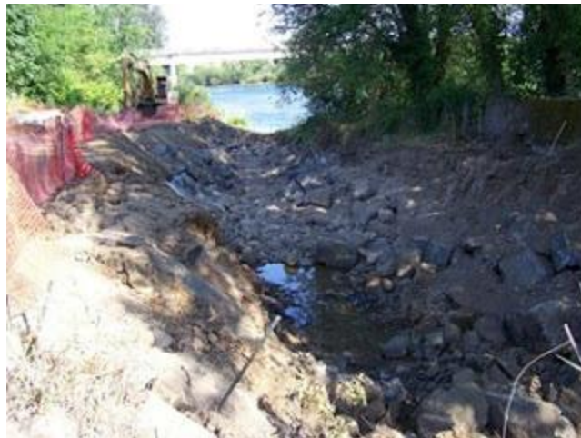
Boulders help habitat in this newly restored stream.
