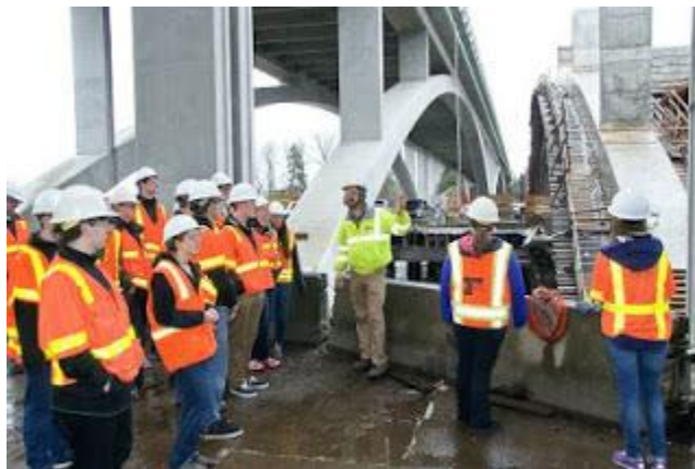
The students learned how the bridge arches and spandrel columns were formed and poured in place to support the roadway deck.
