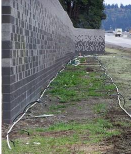
Irrigation lines will help vegetation grow along the new sound wall.
