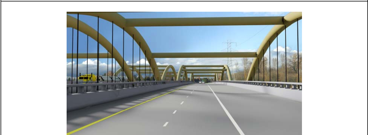
Through Arch Bridge Type
