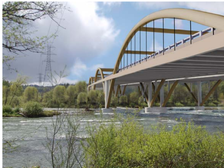
Through Arch Bridge Type
