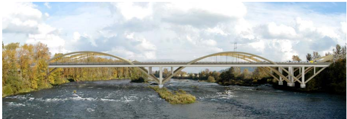
THROUGH ARCH BRIDGE TYPE
