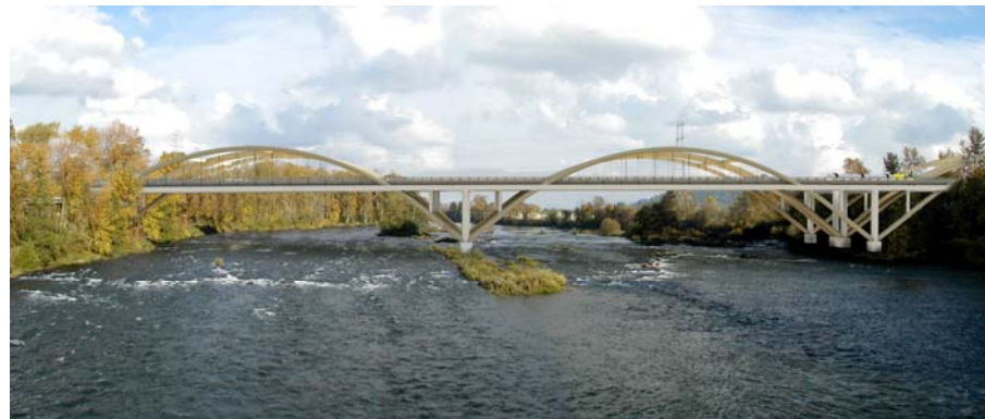
Through Arch Bridge Type
