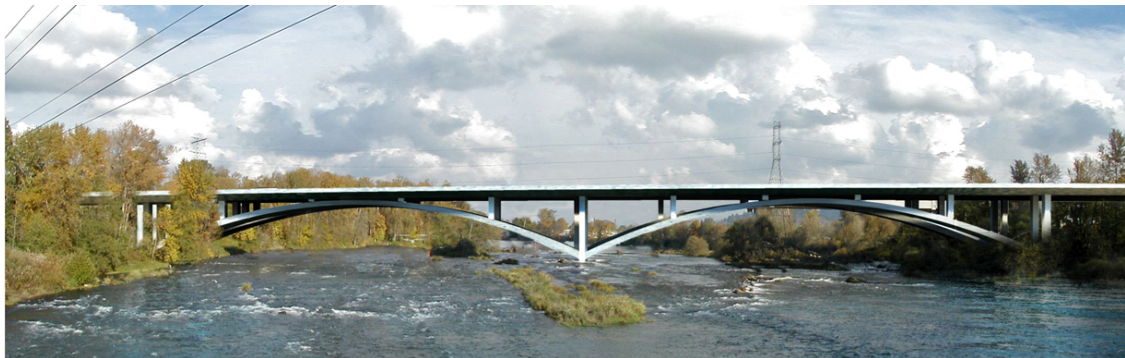
DECK ARCH BRIDGE
