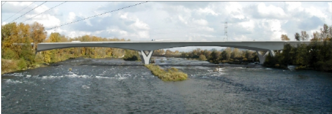
BOX GIRDER BRIDGE
