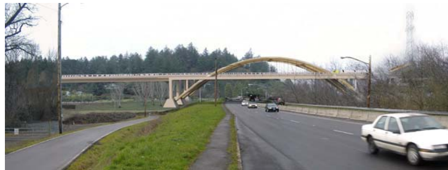
Through Arch Bridge Type
