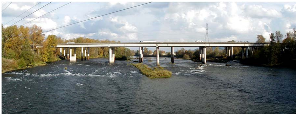
Key View 2: From Knickerbocker bridge looking east.
