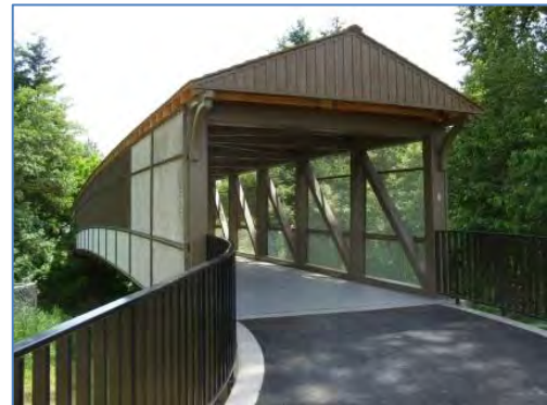
“Pathway to Knowledge” footbridge
