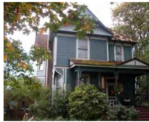
38882 N Main Street Thomas Munker House (ca. 1895)
