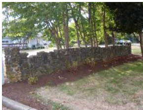
38945 NW 3 rd Avenue Dr. Prill Stone Fence (ca. 1900)
