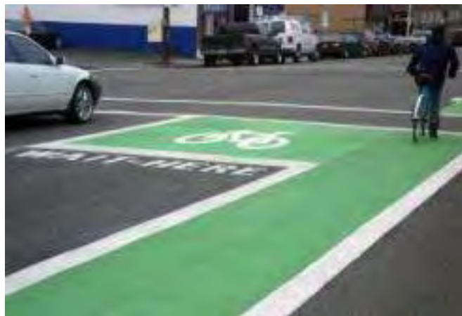
Existing Bicycle Box in Portland
