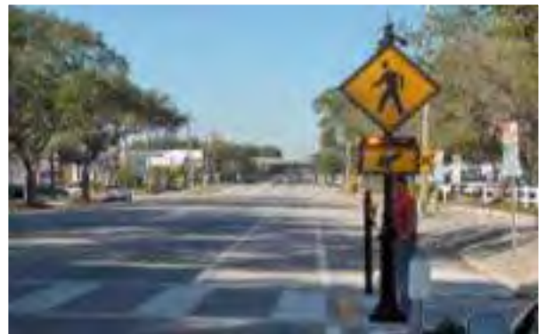
Rectangular Rapid Flashing Beacon
