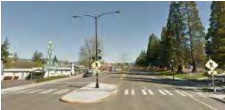
Pedestrian-Activated Crossing in Ashland (Flashing Beacon)
