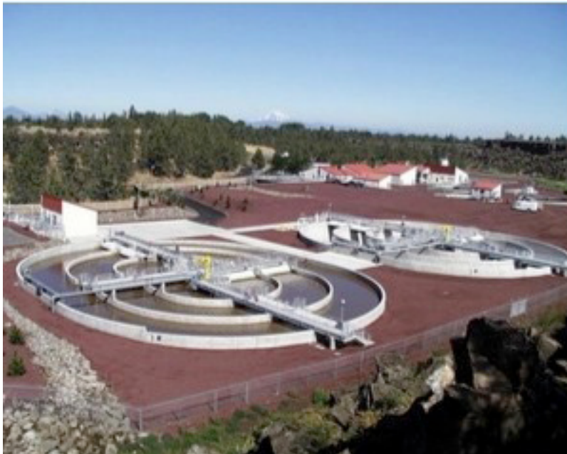
Figure 1: City of Redmond Wastewater Division Facility
