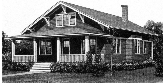
Front gabled roof with hip roofed porch
