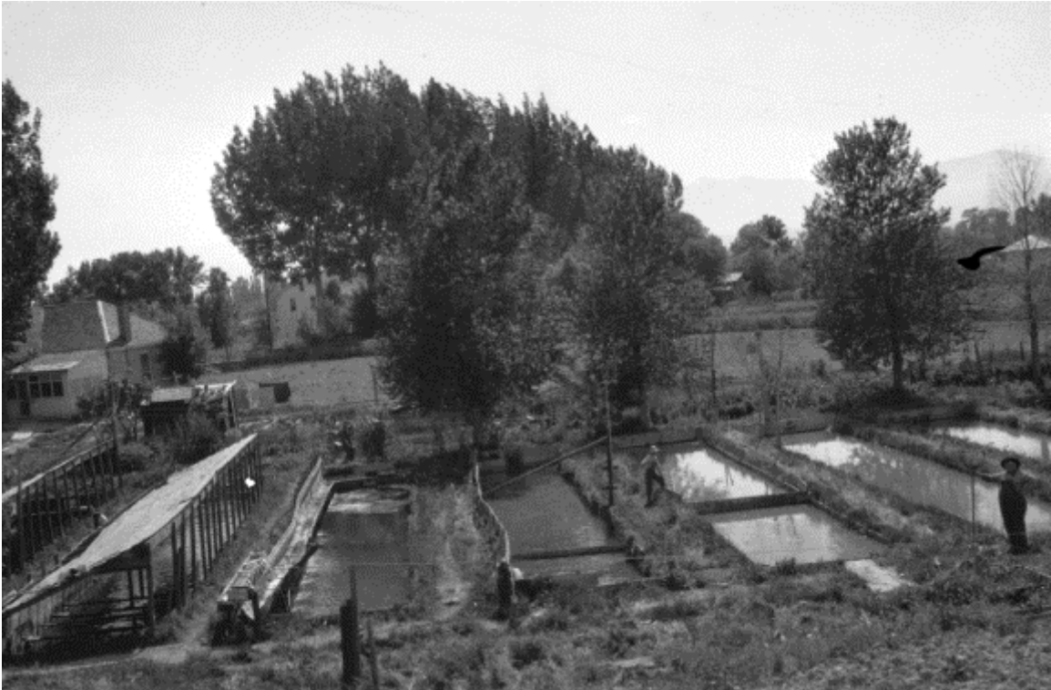
Figure 2.6. Wood-lined, earthen rearing ponds at Millcreek Hatchery, Salt Lake County, Utah c. 1890. Courtesy George M. Ottinger photograph collection, P0123, Special Collections and Archives, University of Utah, J. Willard Marriott Library, Salt Lake City, Utah.
