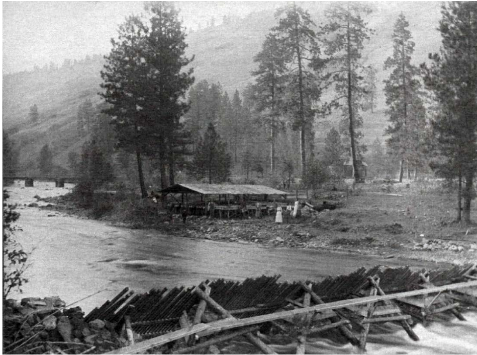
Figure 2.4. Hatchery site including a 'rack' for collecting salmon, the hatchery building with troughs, and a train bridge in the background. The only identifying information locates this scene in Wallowa County c. 1910. Courtesy Oregon Historical Society Research Library, OrHi 3499, Lot 790, Box 19, Folder 14.
