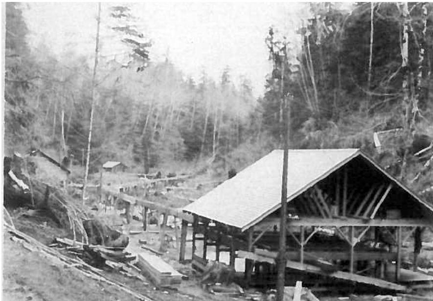
Figure 2.5. Unidentified salmon hatchery building and wood flume c. 1910. Courtesy Oregon Historical Society Research Library, OrHi 3499, Lot 790, Box 19, Folder 14.
