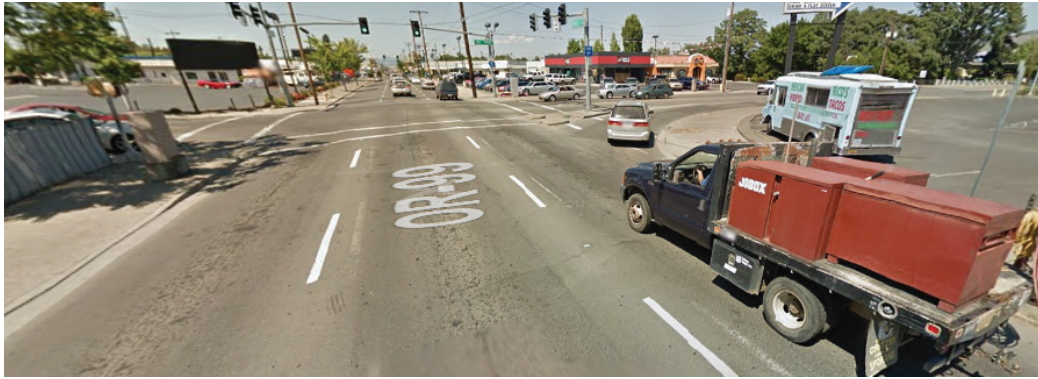
Figure 22: Current conditions on Riverside Avenue/ OR-99.
