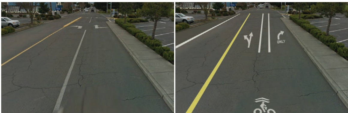
Figure 42: Intersection at Medford Center Road and Jackson Street.
