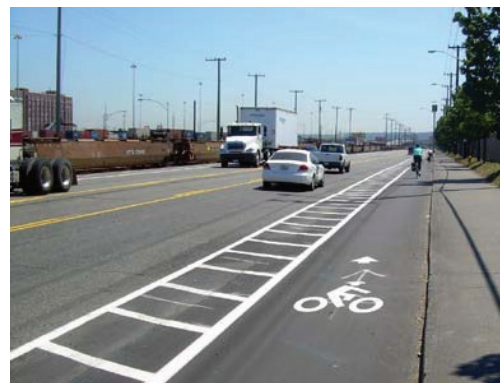
Figure 37: Hatch markings can act as sufficient and more cost-effective buffer to separate bike lanes from vehicle traffic. Credit: Seattle Department of Transportation.
