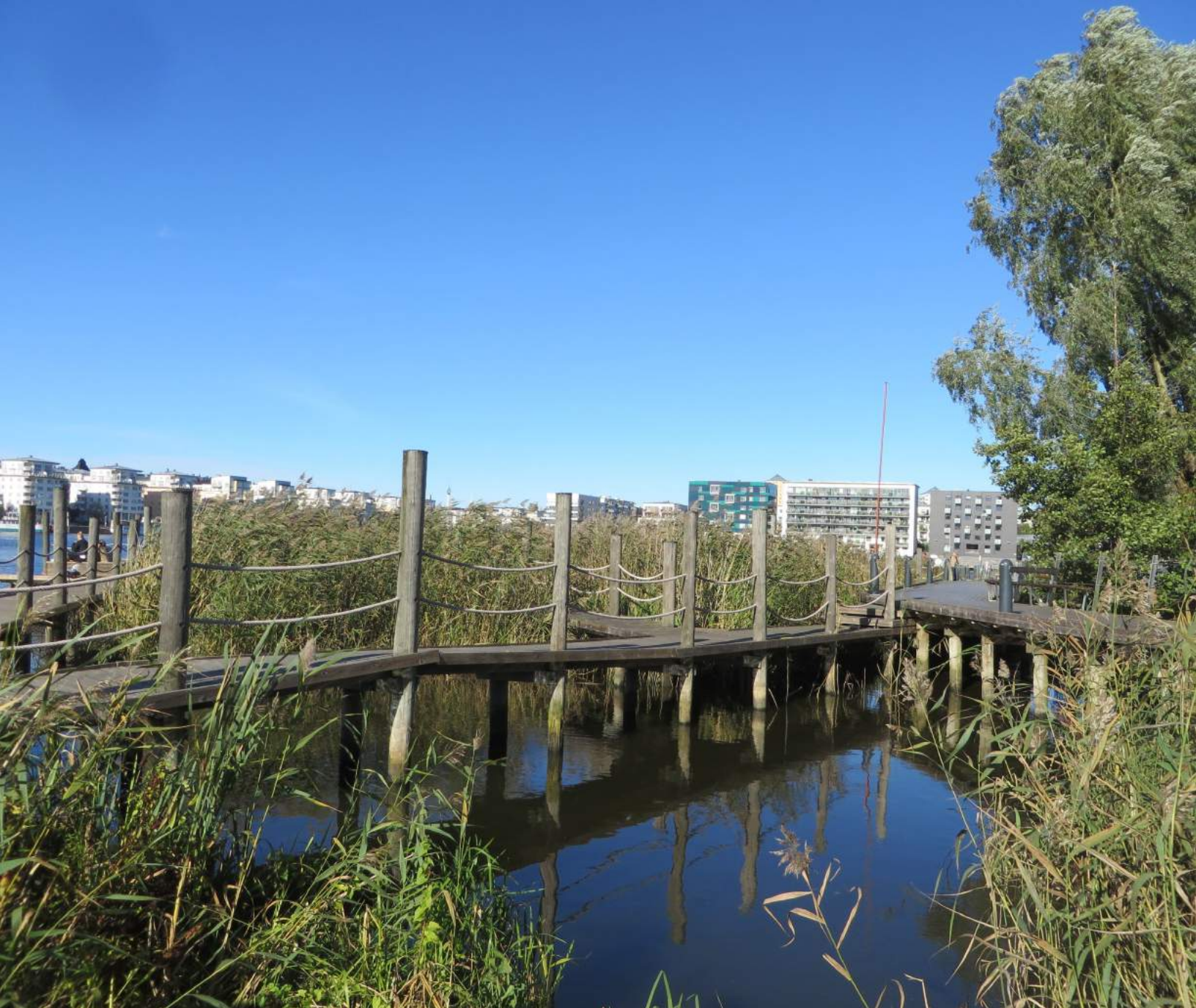
Adapt parks to their location when possible; this system of boardwalks laces among grasses in a harbor south of Stockholm, Sweden.
