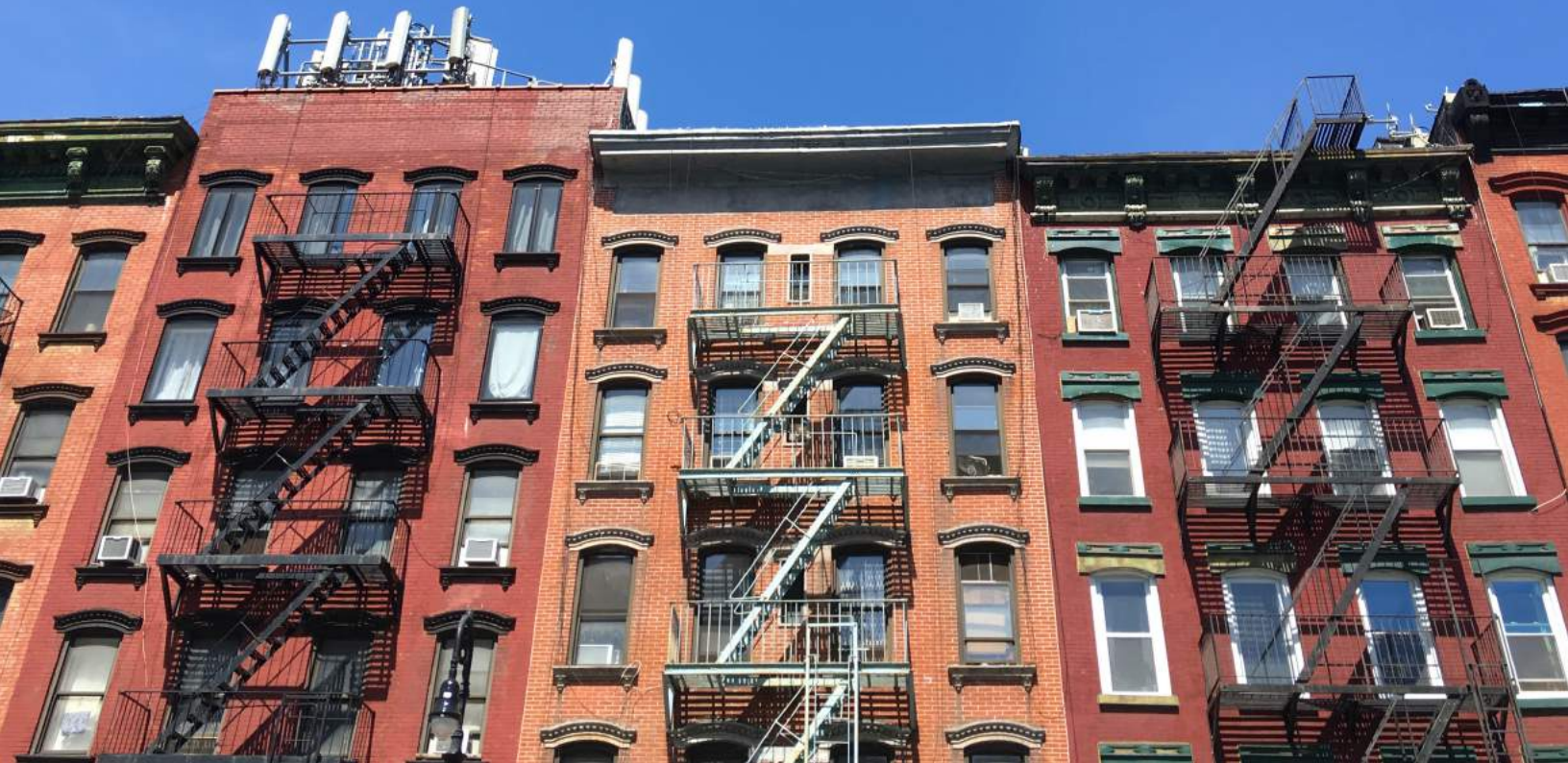
Abutting buildings are the ultimate example of infill, here in New York City.
