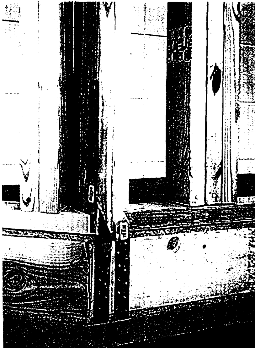
Figure 6-3, Truss to SIP Connection using Metal Straps
