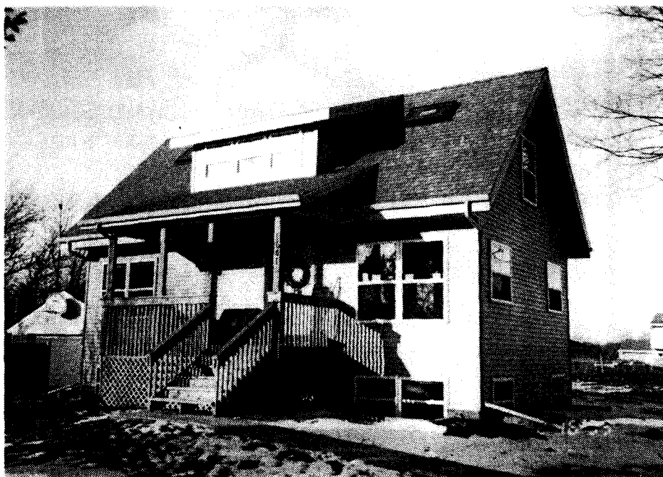
Figure 8-2, Front of READ Project House, East Lansing, MI
