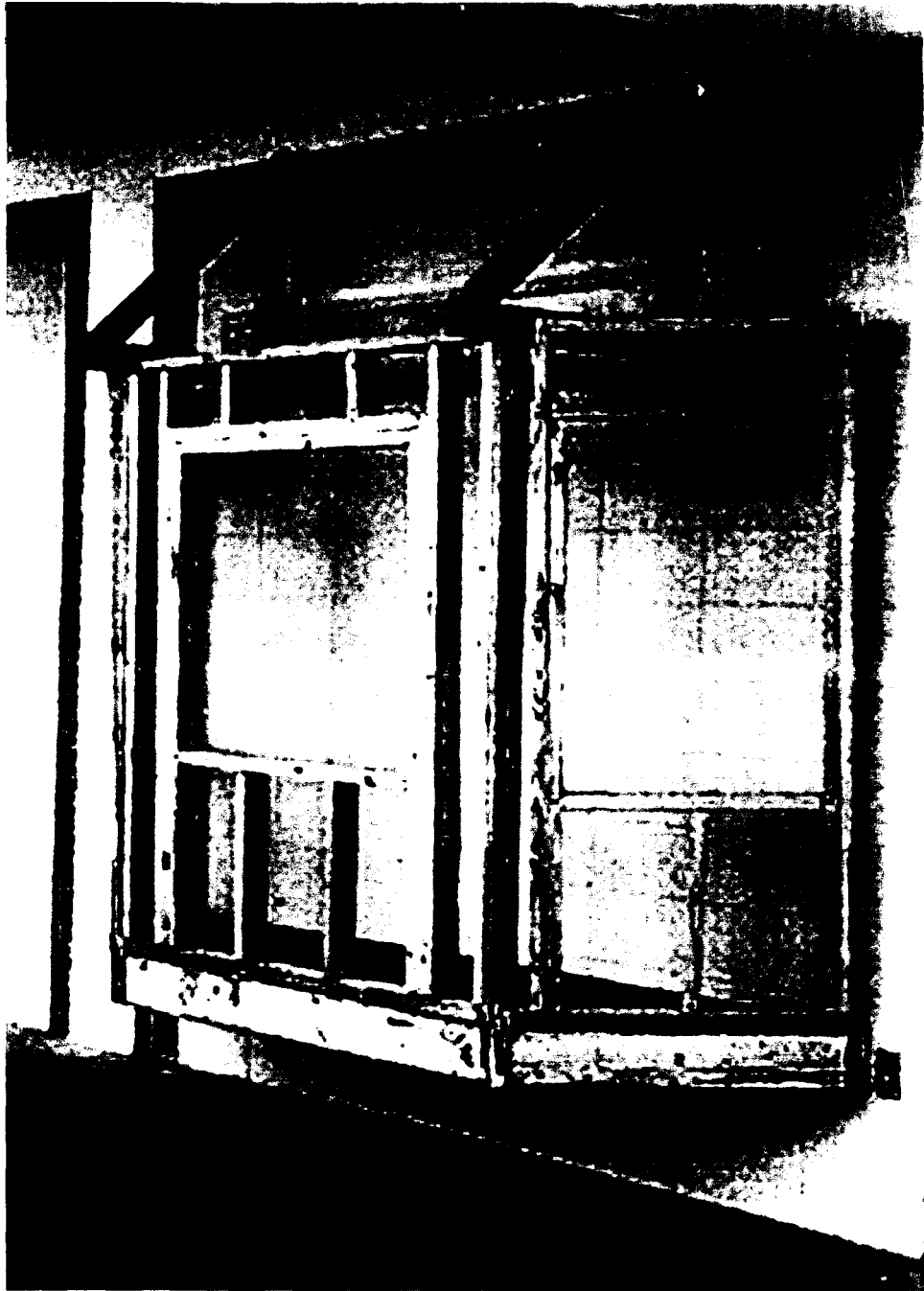
Figure 6-5, Completed Bay Window Prototype
