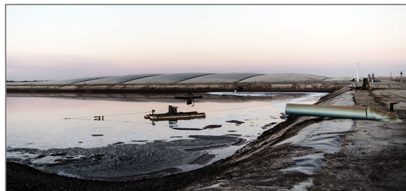
FIGURE 2. UNCOVERED MANURE LAGOON.
