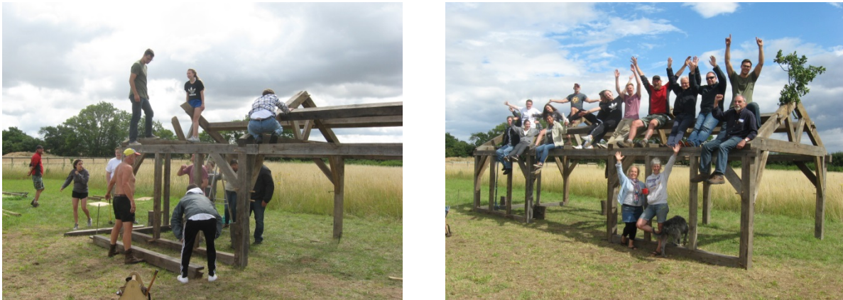
Fig. 2. Students constructing a heavy timber frame in Suffolk, UK (2017)
