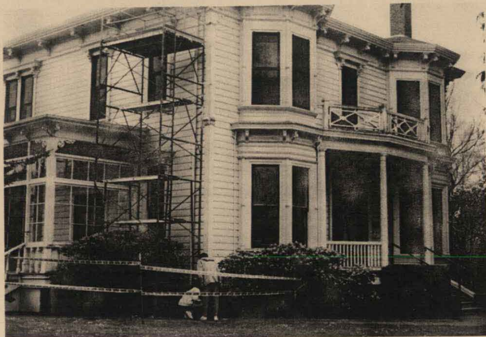
The Collier House, Northeast Corner, 1990.
