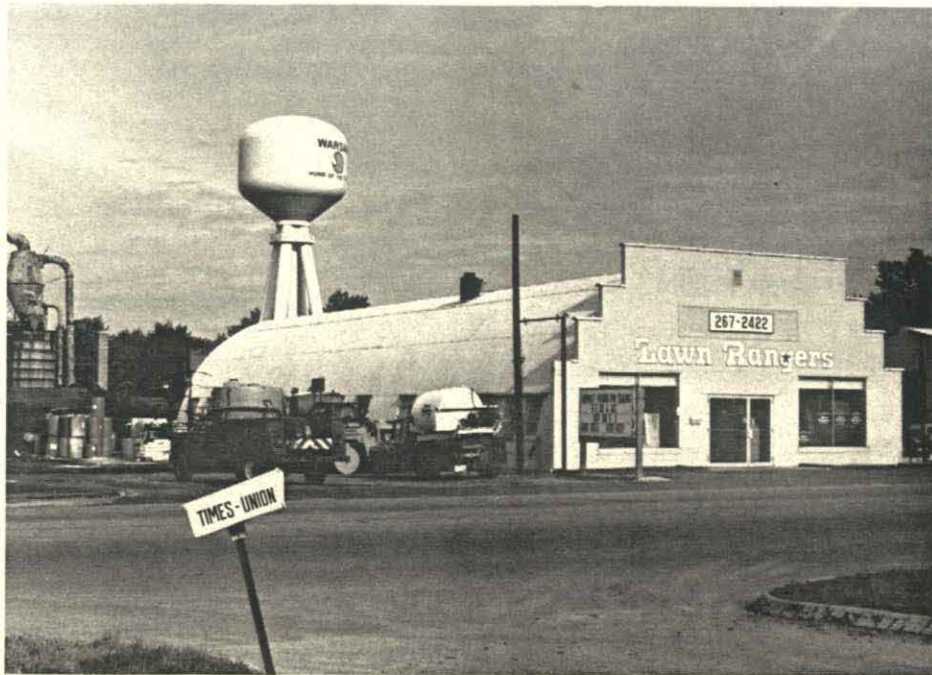
A typical model "40" quonset hut with a 1940's facade. This particular hut is located in Warsaw, Indiana, but the form can be found on approach strips and in towns all over America, with many facade variations.
