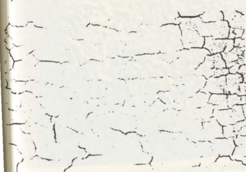
Fig. 5 Crazing—or surface cracking—is an exterior surface condition which can be successfully treated by sanding and painting. Photo: Courtesy, National Decorating Products Association.
