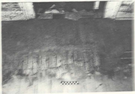
Fig. 21. Patch of false graining on parlor floor.
