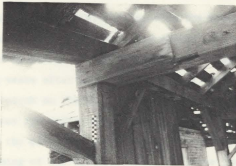
Fig. 5. Southeast end of woodshed. Note that beam only butts up to post.
