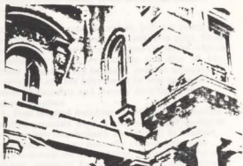
Illus. 9. Simple solutions should not be overlooked when materials are no longer available. In the case of the Morse-Libby Mansion (1859), Portland, ME, the deteriorated brownstone porch beam was replaced with a carved wooden beam painted with sand-impregnated paint. Photo: Stephen Sewall.
