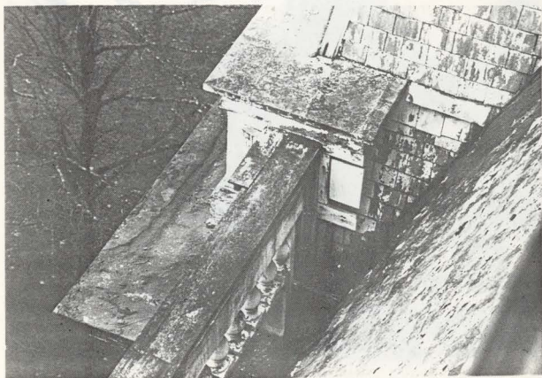
PHOTOGRAPH 3. North-Elevation Balustrade as Viewed From the Main Roof: Existing Condition
