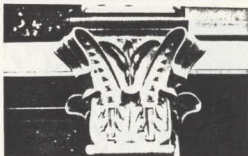
Close-up detail showing the crisp casting in aluminum of this 19th-century replica column and capital for a storefront. Photo: Sharon C. Park, AIA.
