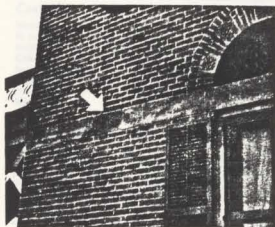
Illus. 21. Change of color over time is one of the greatest problems of synthetic substitute materials used outdoors. Ultra-violet light can cause materials to change color over time, some will lighten and others will darken. In this photograph, the synthetic patching material to the sandstone bonding to the left of the window has aged to a darker color. Photos: Sharon C. Park, AIA.
