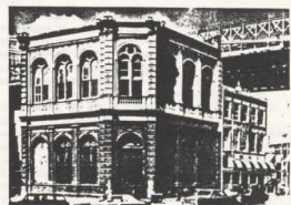
Illus. 4. The 19th century also produced a variety of metal products used in imitation of other materials. In this case, the entire exterior of the Long Island Safety Drydock Company is cast-iron representing stone. Photo: Basket Lagan, Friends of Cast Iron Architecture.
