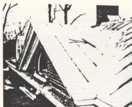
Illus. 12. Substitute materials may be considered when the original materials have not performed well. For example, early sheet metals used for roofing, such as tinplate, were reasonably durable, but the modern equivalent, terne-coated steel, is subject to corrosion once the thin tin plating is damaged. Terne-coated stainless steel or lead-coated copper (shown here) are now used as substitutes. Photo: John G. Waite.
