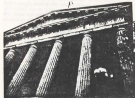
Illus. 13. Code-related changes are of concern in historic preservation projects because the integrity of the historic resource may be irretrievably affected. In the case of the Old San Francisco Hotel, the fiberglass cornice was used to bring the building into seismic conformance. The original cornice was deteriorated, and the replacement (1982) was limited to the projecting pediment. The historic stone fascia was retained as were the stone columns. The limited replacement of deteriorated material did not jeopardize the integrity of the building. Photo: Walter M. Sonthener.
