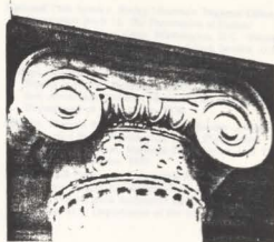
This replica column capital was made using epoxy resins poured into a mold taken from the building. The historic wooden column shaft was repaired during the restoration. Photo: Courtesy Dell Corporation.
