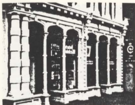
Illus. 11. The unavailability of historic craft techniques is another reason to consider substitute materials. The original first floor cast iron front of the Grand Opera House, Wilmington, DE, was missing; the expedient reproduction in cast aluminum was possible because artisans working in this medium were available. Photo: John G. Waite.
