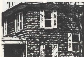
Illus. 3. Casting concrete to represent quarried stone was a popular late 19th-century technique seen in this circa 1910 mail-order house. While most components were delivered by rail, the foundations and exterior masonry were completed by local craftsmen. Photo: Sharon C. Park, AIA.
