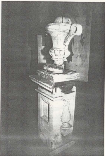
FIGURE 16. Remains of the Morris M. Marks House Front-Porch Roof-Line Urn/Balustrade Stored in the Attic: 1988 View (Note the broken base of the urn.)
