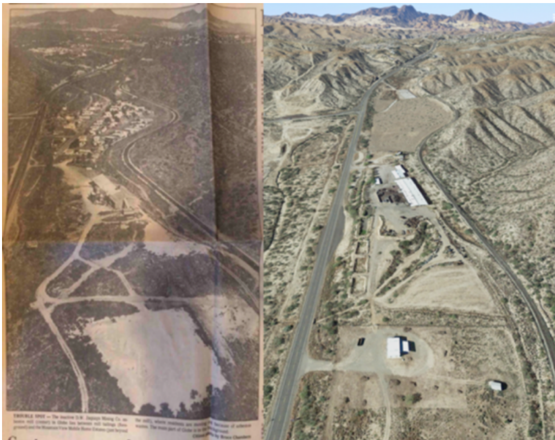
Figure 7.1. Left: Metate Asbestos mill in center with Mountain View Mobile Home Park behind it. Right: The long, white-roofed building in the center is Chem Metals, Inc., with the site of the former Mountain View Mobile Home Park behind it. Looking west toward Globe. Sources: Tucson Citizen , June 17, 1983, and Google Maps.
