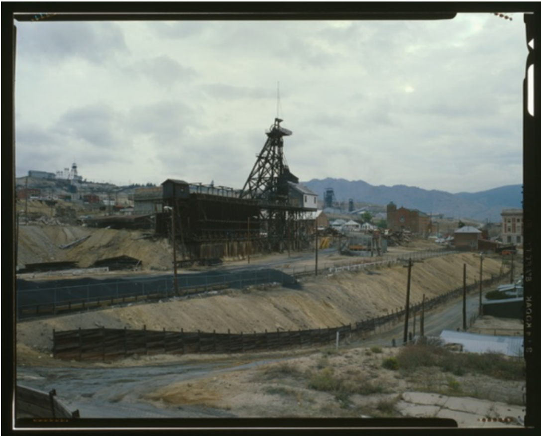
Figure 7.5. The Original Mine, Butte, Montana. The 1980 photograph for the Historic American Engineering Record depicts a mining headframe in the center of town, surrounded by waste rock piles and crumbling mine structures. Source: Library of Congress.
