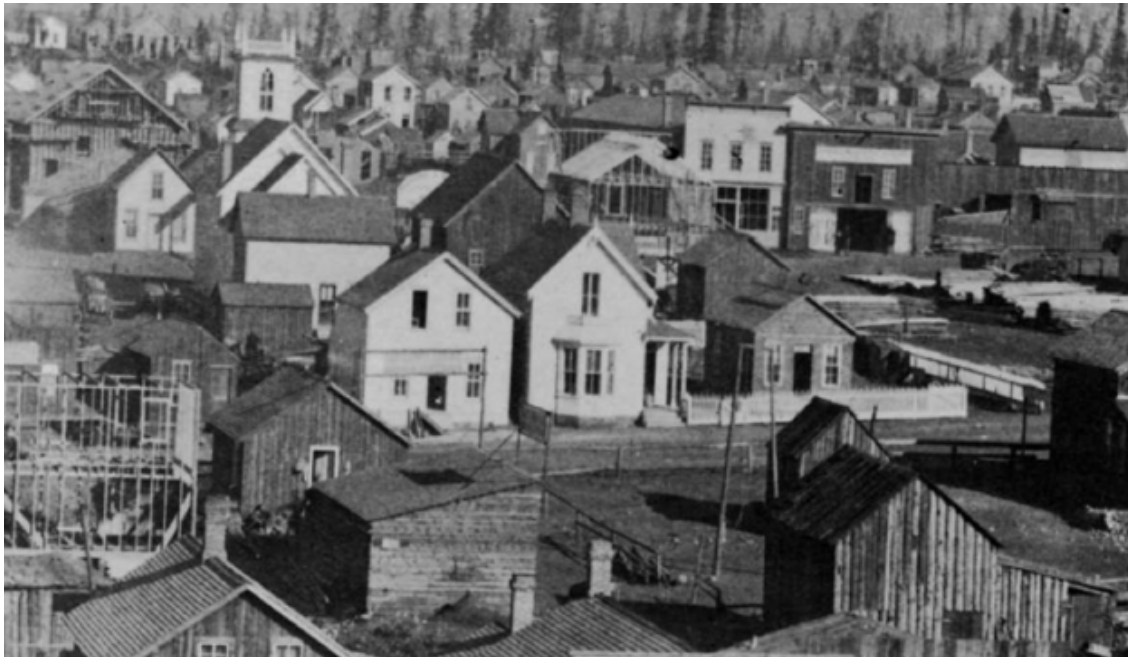
Figure 3.1. The Tabor house at its 116 East Fifth Street address, c. 1879. The Tabor Home is the white one and a half story structure with bay window (center). Photo by George D. Wakely. From Denver Public Library's Western History and Genealogy Department, Call number X-6301.
