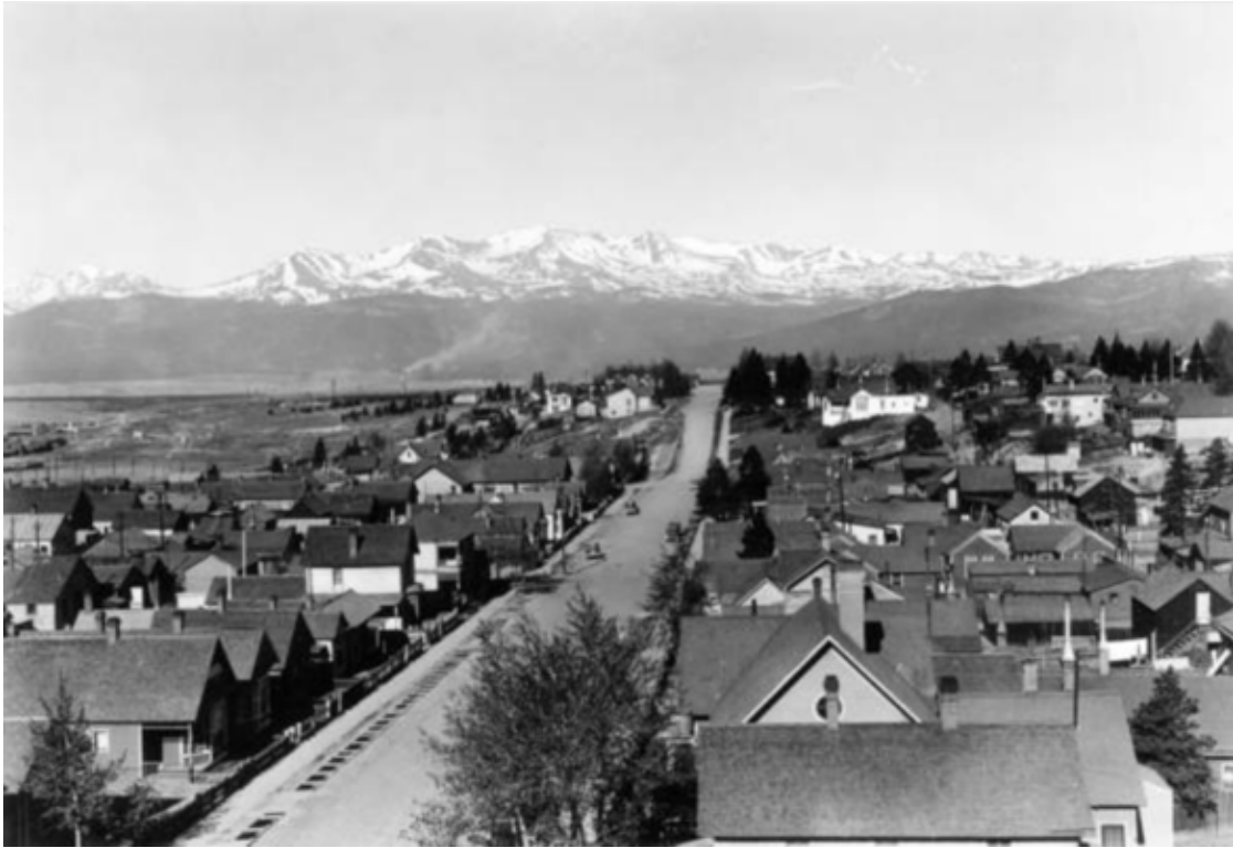
Figure 4.11. 1920s image of Leadville, looking west along Eighth Street. This was a fairly well-off neighborhood and shows that many of the houses had shingled roofs. The Larsh/Mascarenas home would be just beyond the left frame of this image. Source: Call Number CHS.X5369, http://digital.denverlibrary.org/cdm/search/searchterm/CHS.X5369 Denver Public Library Western History and Genealogy, Denver, Colorado.
