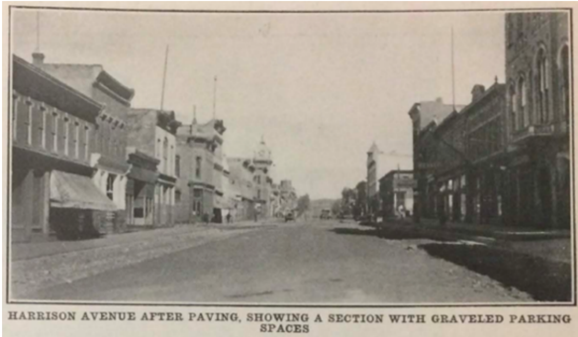
Figure 4.9. Harrison Avenue in Leadville after 1930 paving project, looking north. Note the contrast between muddy and rutted Figure 4.8 to smooth and dry in Figure 4.9. From J.D. Wilder, "Building City Streets 10,000 Feet Above Sea Level," American City 42 (January 1930): 123.
