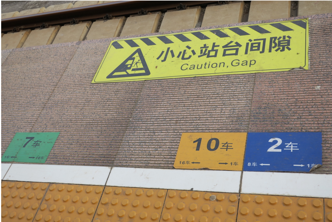
Figure 4.21. The colored plaques embedded in platforms serving HSR trains facilitate boarding by showing passengers where the doors to the train will be located once it arrives. When the train misses its mark, passengers and personnel have to scramble.
