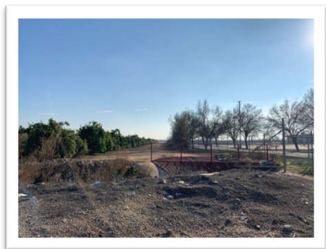
Manning Avenue at Tobu Avenue (south); Image Source: Jenna Chilingierian
