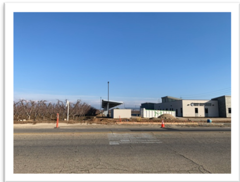
Buttonwillow Avenue at Manning Avenue (east); Image Source: Jenna Chilingirian
