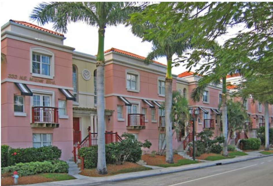
Image 7.11 Mizner Park's neighbors look on to these town homes, oriented wide and shallow to hide a parking garage.
