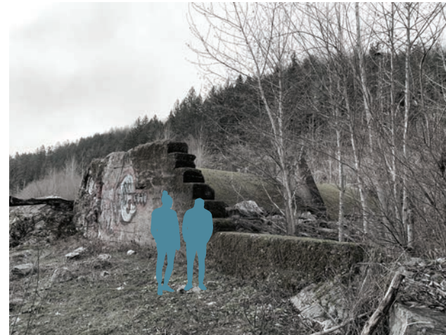
Figure 5.2: "Leave-as is," demonstrated at Savage Rapids Dam Trace #5, the Stepped Buttress Wall
