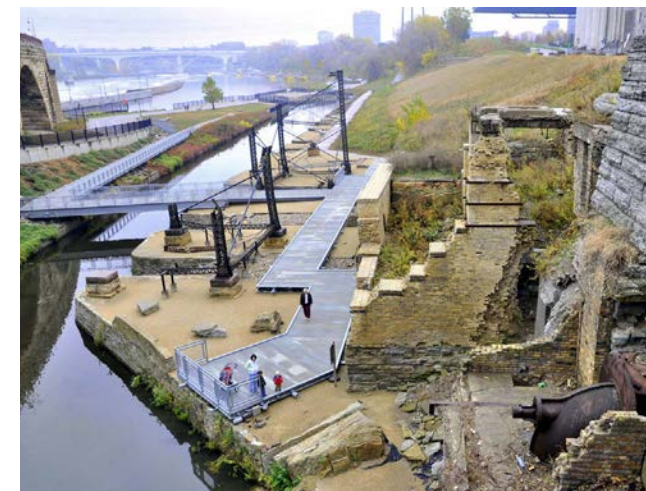
Figure 3.9: Concrete and Steel Walkway Providing Access to Ruins, from: Rant Lifestyle, http://www.rantlifestyle.com/2014/05/08/top-10-landmarks-in-minneapolis/ , accessed May 1, 2021
