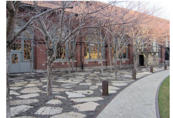
Figure 3.3: Recycled Pavement from Site Demolition in Planters, from: D.I.R.T. Studio, http://dirtstudio.com/#urbndd , accessed May 1, 2021
