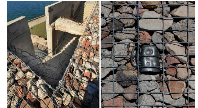
Figure 3.6: Historic Artifacts Found During Demolition Encased in Rubble Gabions, from: McGregor Coxall, https://mcgregorcoxall.com/project-detail/125 , accessed May 1, 2021
