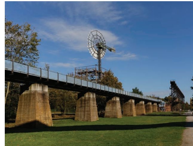
Figure 3.12: Steel Walkway Built Over Remnant Railway Pilings, from: Latz + Partner, https://www.latzundpartner.de/en/projekte/postindustrielle-landschaften/duisburg-nord-bahnpark/ , accessed May 1, 2021
