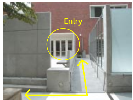
Recommended: Ramp design providing easy access to building entrance without negatively impacting the character of the building (Portland Art Museum)
