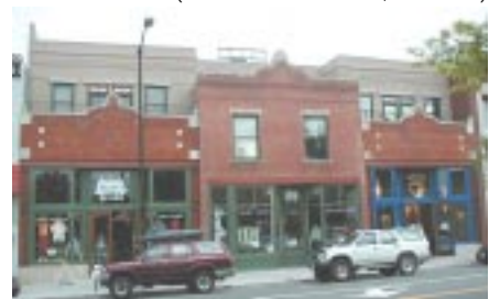
Recommended: Addition of second story building is set back from the historic facade (Boulder, CO)
