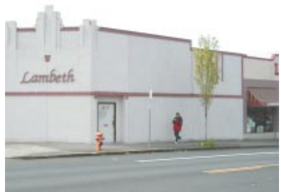
Not Recommended: "Dead edge" created by providing no window openings or building articulation along the lower 15' of the building (N Denver and Schofield, Portland)
