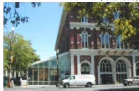
Not Recommended: Addition does not relate well in form, massing or materials (SW 2nd and Ankeny, Portland)
