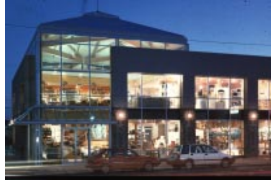
Recommended: Transparency of facade fosters interaction between the public and private realm (NE Broadway and 15th, Portland)
