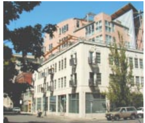
Not Recommended: Contemporary addition on top of historic building contrasts too greatly in form, color and materials with the existing building below. (NW 8th and Flanders, Portland)
