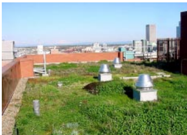
Recommended: Roof that includes landscaping to filter rainwater (SW 12th and Clay, Portland)
