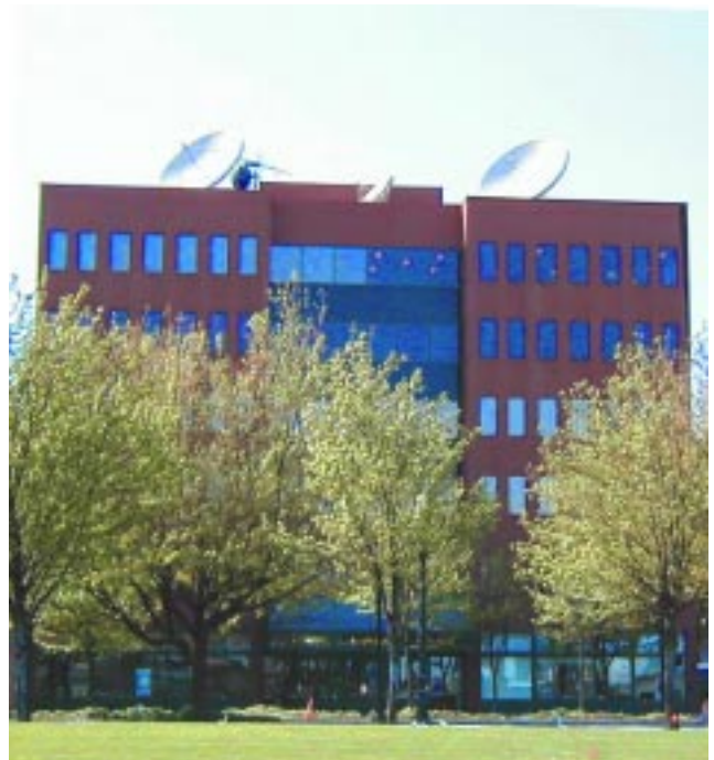
Not Recommended: Rooftop equipment visible and not integrated into building design (SW 2nd and Stark, Portland)
