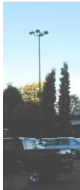
Not Recommended: Overscaled, utilitarian lights in parking lots (SW 2nd and Alder, Portland)
