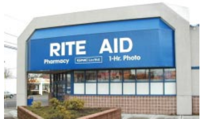
Not Recommended: Vinyl awning sign (N Lombard and N Denver, Portland)
