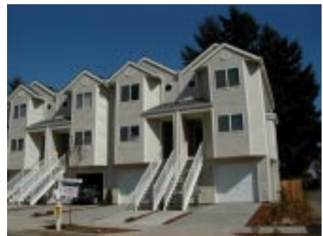
Not Recommended: Entry doors too high above street level (East Burnside and 104th, Portland)
