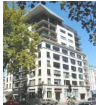
Recommended: Contemporary additions on rooftops can be compatible with the historic building if the historic facades are left intact (NW 8th and Everett, Portland)
