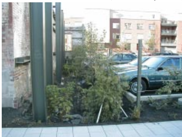
Recommended: Polluted water runoff from parking lot is mitigated by a landscaped swale (NW 10th and Irving, Portland)
