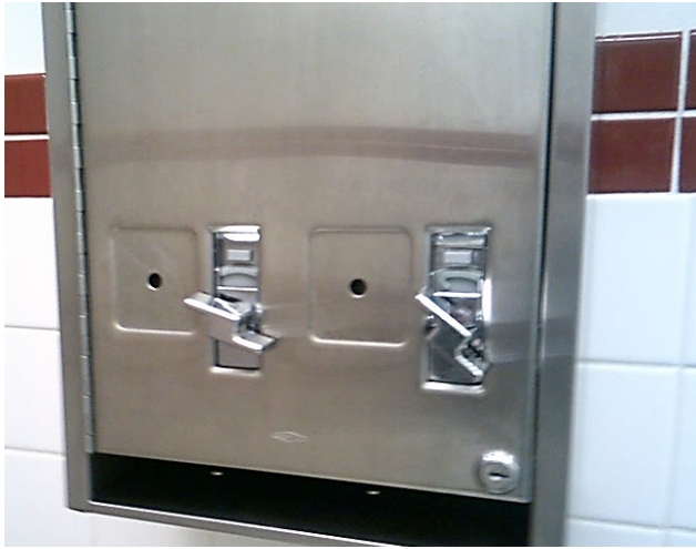
Figure 19: The broken tampon dispenser at the field site.
